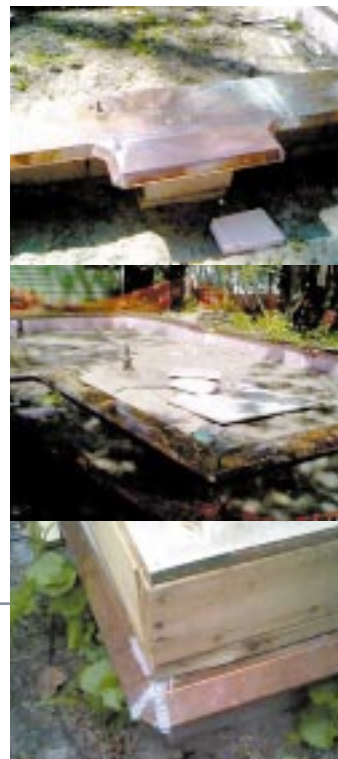
PHOTO 4,5 and 6: Termite shields, or sheet metal barriers, are installed between the top of the foundation and the sill plate. By projecting out and down at a 45 degree angle, the barriers force termites to tube around them for easier detection. [Photos: Tim Myles, University of Toronto]
