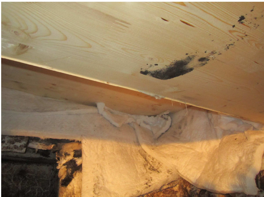
Exposed Side Prior to the Fire Test
