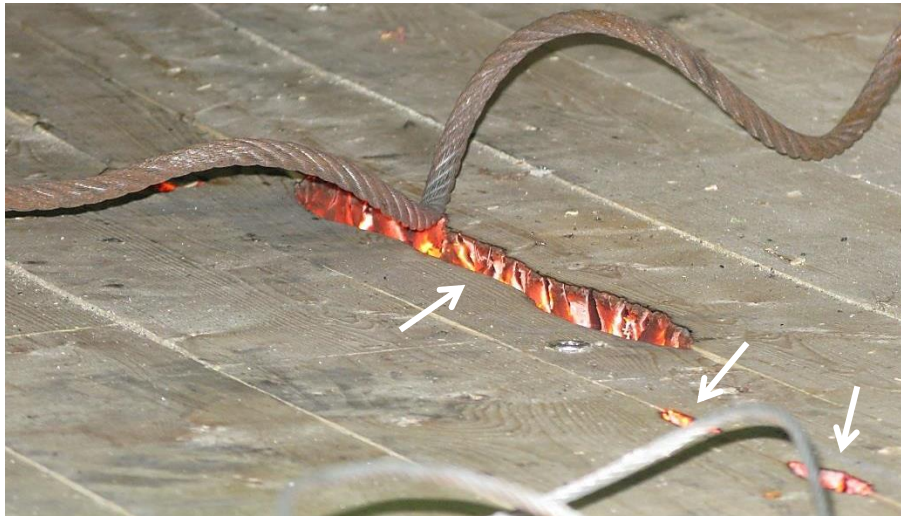
Figure 7. Failure of the 3-ply half-lapped joint
