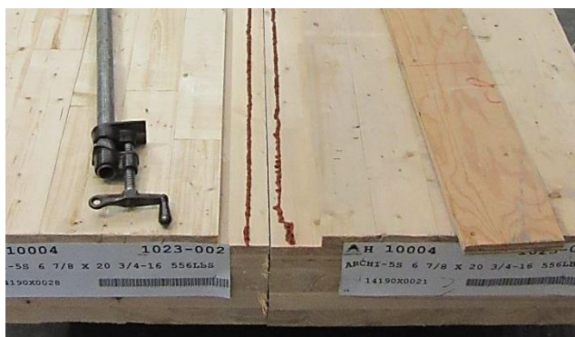
c) Single surface spline
