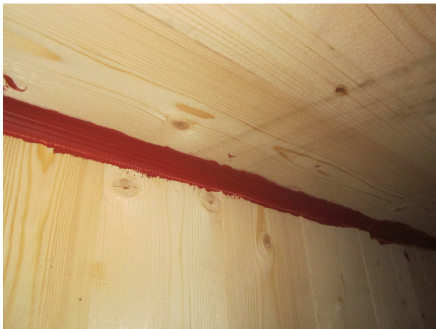
Exposed Side Prior to the Fire Test
