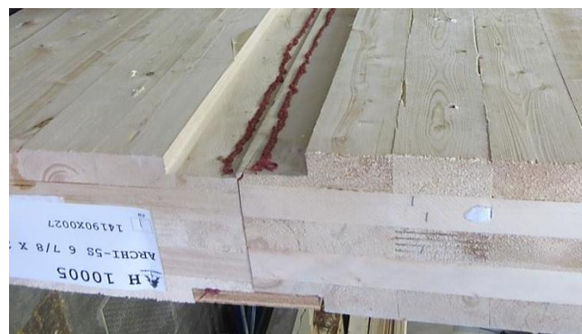
d) Double surface spline
