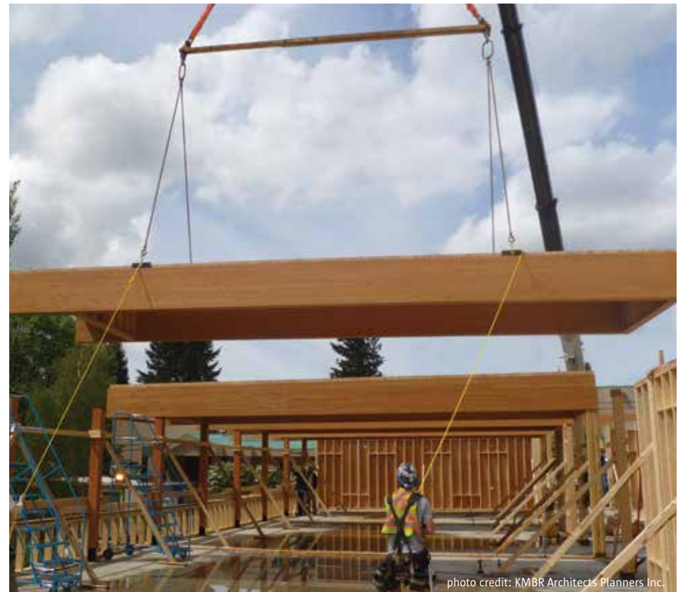
Figure 5.4: Surrey Christian School: Installation of NLT roof panels
