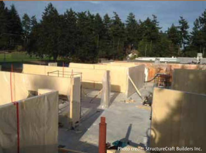
Figure 4.5: Cordova Bay: Installation of CLT wall panels
