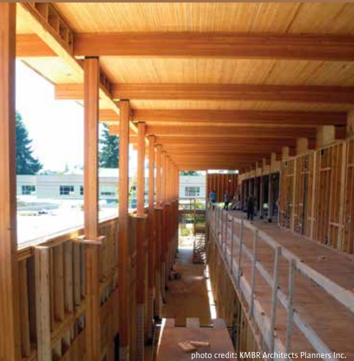
Figure 5.2: Surrey Christian School: View of post-and-beam structure at the atrium
