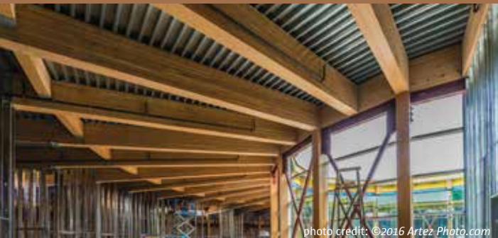
Figure 3.9: Wellington Secondary: Radial post-and-beam structure of Block F
