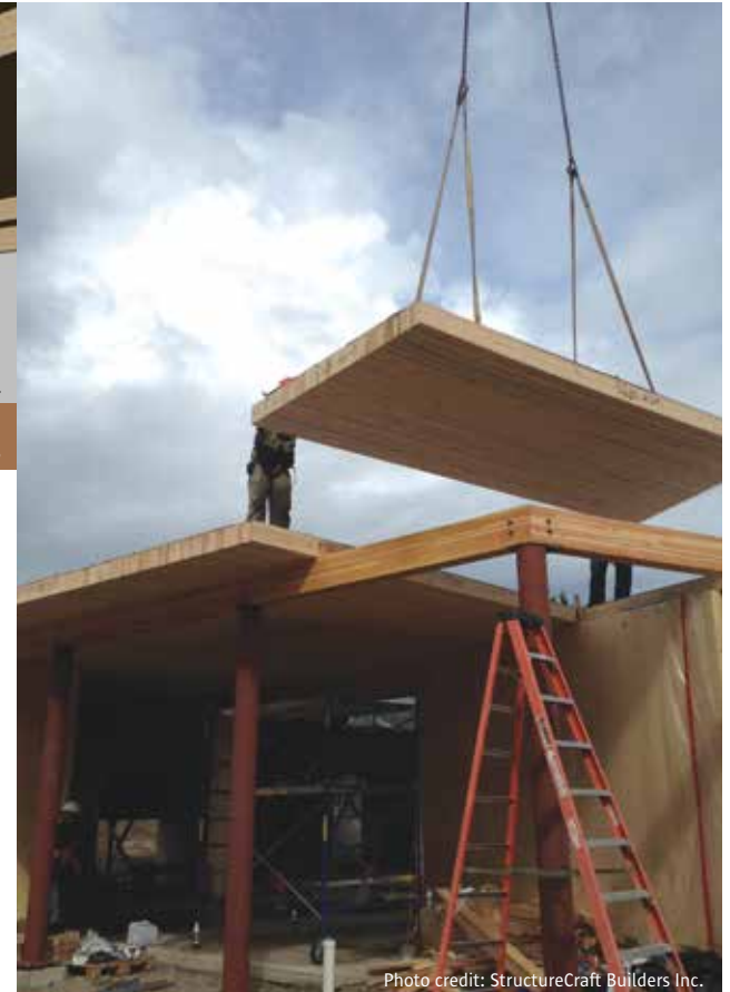
Figure 4.9: Cordova Bay: Installation of NLT roof panels
