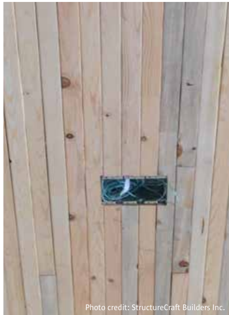
Figure 4.11: Cordova Bay: Service chase in NLT panel with cover strip installed
