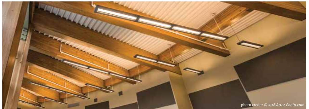
Figure 3.4: Wellington Secondary: New structural members in Block F
