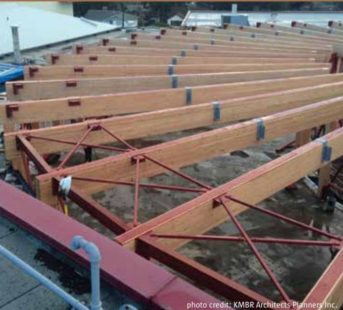
Figure 3.8: Wellington Secondary: Roof top view of drag rings for load transfer
