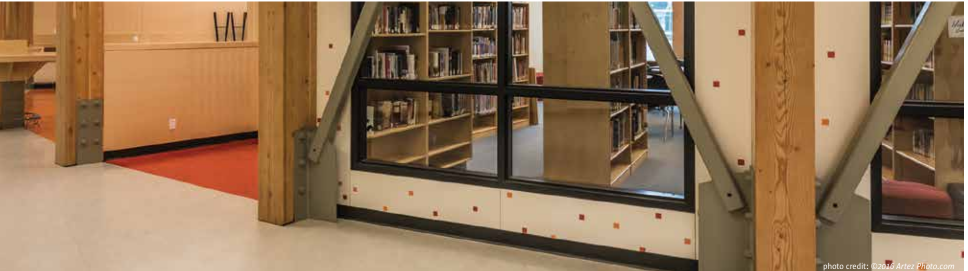
Figure 3.13: Wellington Secondary: New glulam columns fitted with seismic cross-bracing
