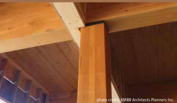
Figure 5.7: Surrey Christian School: Detail of roof beam-to-column connection
