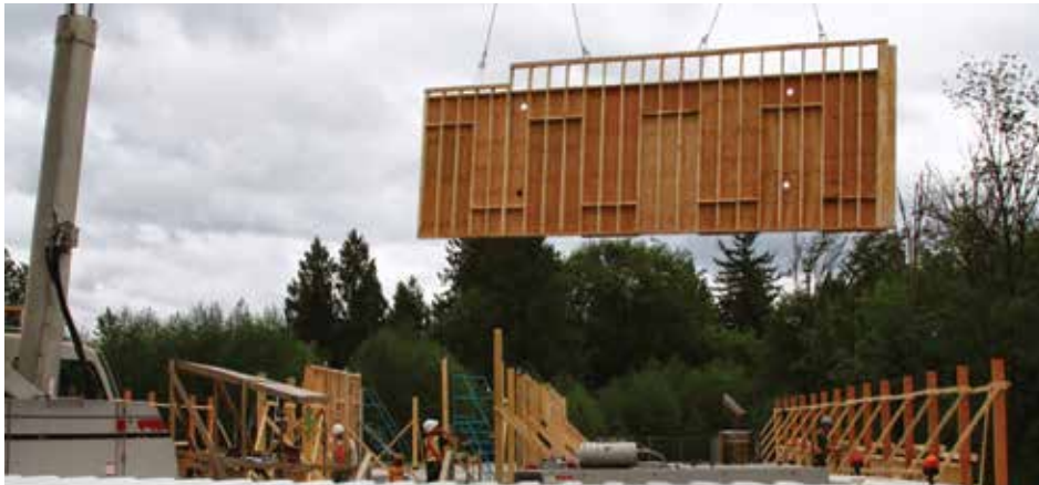
Figure 5.8: Surrey Christian School: Installation of prefabricated light wood-frame shear walls
