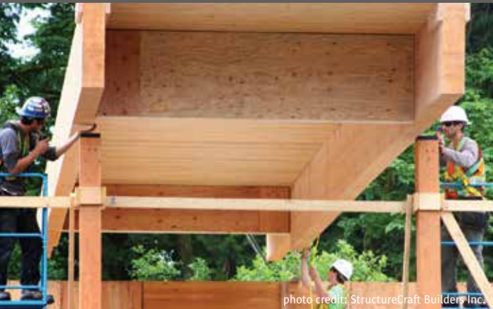
photo credit: StructureCraft Builders Inc. Figure 5.5: Surrey Christian School: Installation of NLT roof panels
