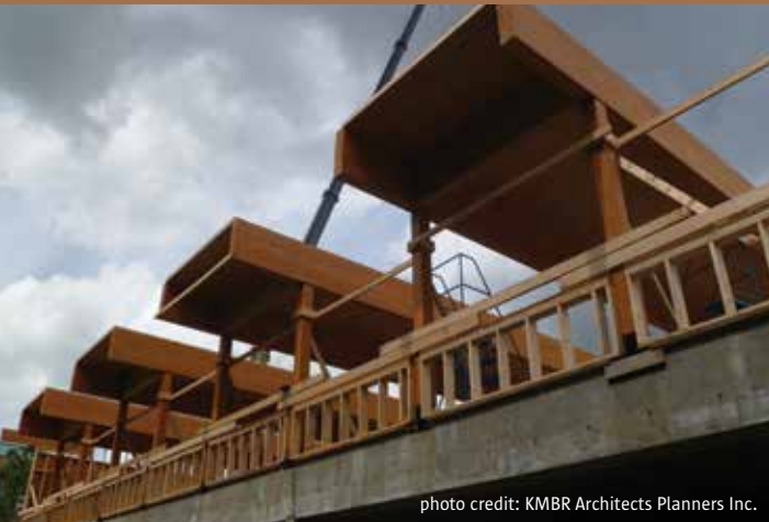
Figure 5.6: Surrey Christian School: Primary roof panels installed in alternate bays leaving gaps for infill panels
