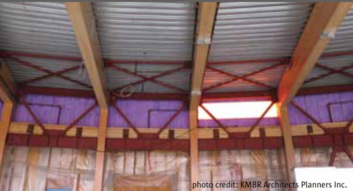
Figure 3.7: Wellington Secondary: Interior view of drag rings for load transfer
