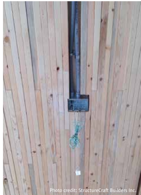
Figure 4.10: Cordova Bay: Service chase cut in NLT panel
