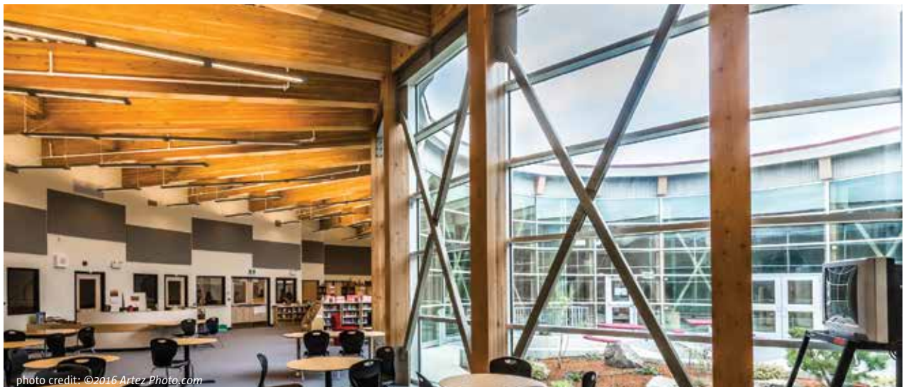
Figure 3.10: Wellington Secondary: Cross-bracing around the perimeter of the courtyard provides lateral stability
