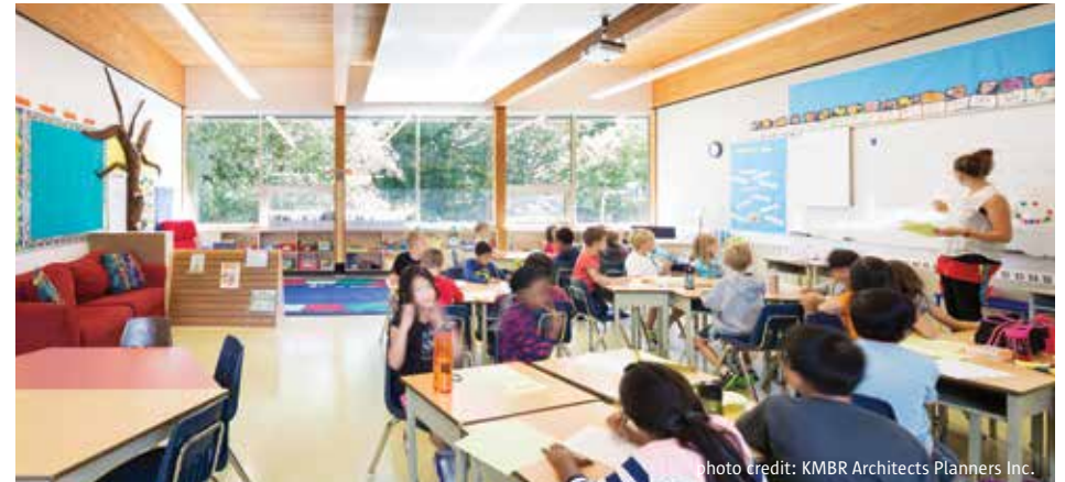
Figure 5.10: Surrey Christian School: A suspended ceiling conceals services in the central bay of each classroom, enabling the NLT panels on either side to remain exposed
