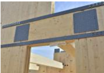
Steel stability plates.
