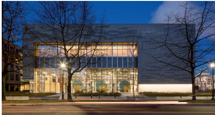
UBC Campus Energy Centre Vancouver, BC
