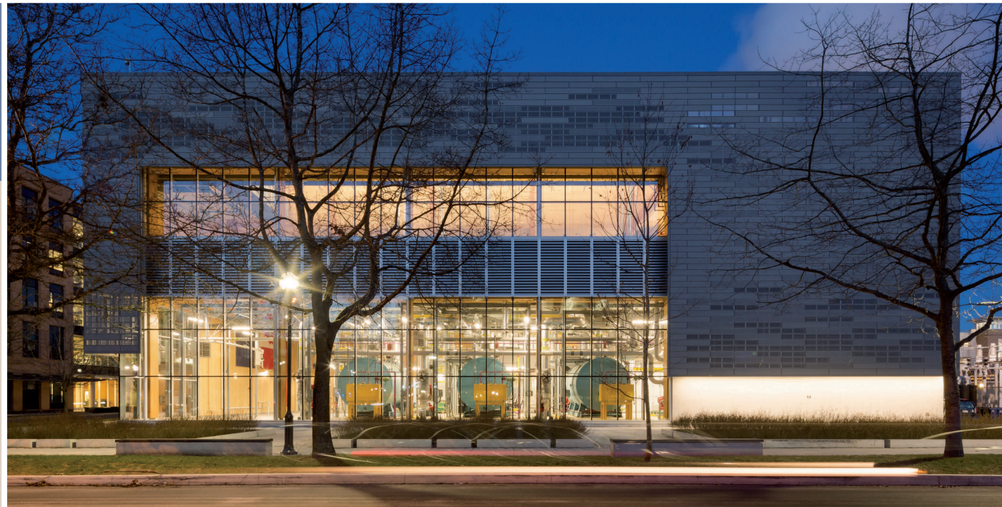
Fig.3.1: UBC Campus Energy Centre
