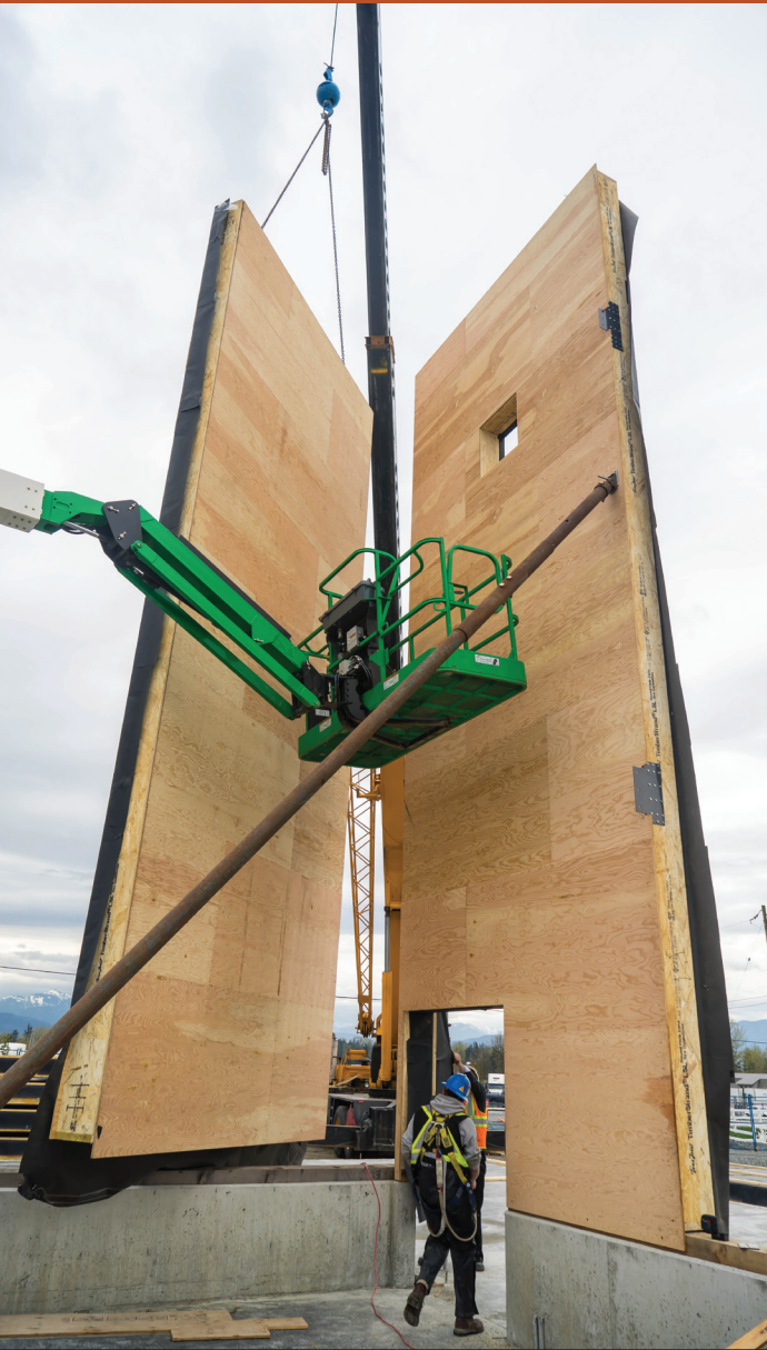
Fig. 4.5: Wall panel being placed
