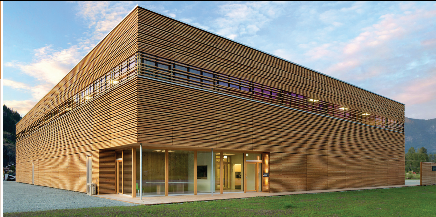
Fig. 2.1: BC Passive House Factory
