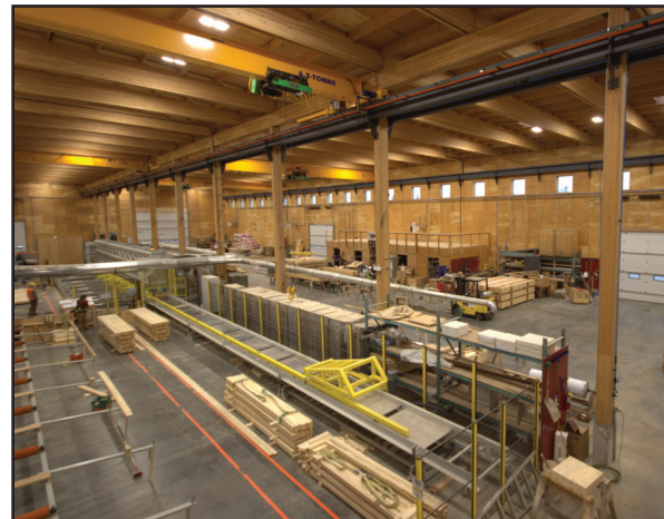
Fig. 4.3: Interior of factory showing central line of columns
