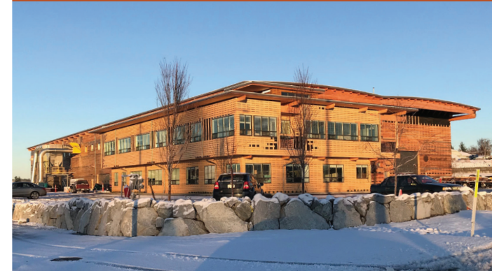
Fig. 4.1: Although they appear to be a single building, the office and factory areas are structurally distinct
