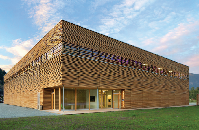
Fig. 2.1: The rectangular volume of the building is clad entirely in wood
