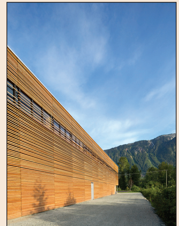
Fig. 2.14: The wood cladding is left unfinished, and will weather to a grey colour over time
