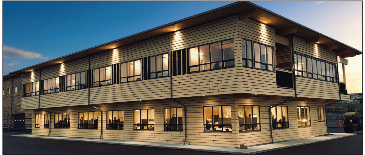
Fig. 4.13: Exterior of office building
