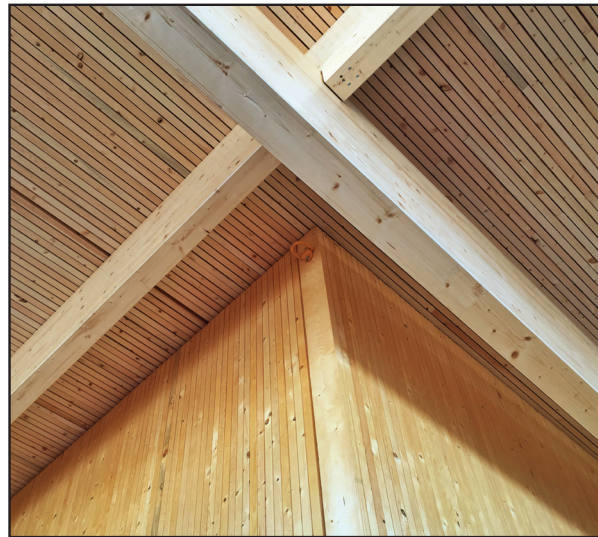
Fig. 4.14: DLT panels in the office area
