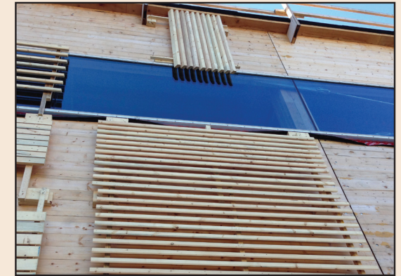
Fig. 2.13: Prefabricated wall panel with fir and larch slats
