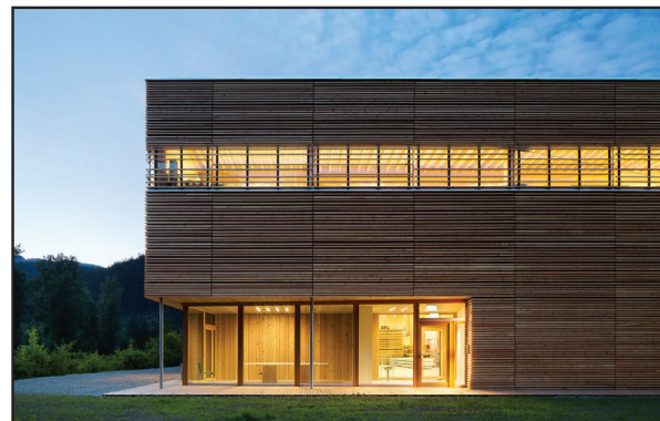
Fig. 2.3: The showroom and office areas are constructed to the Passive House Standard
