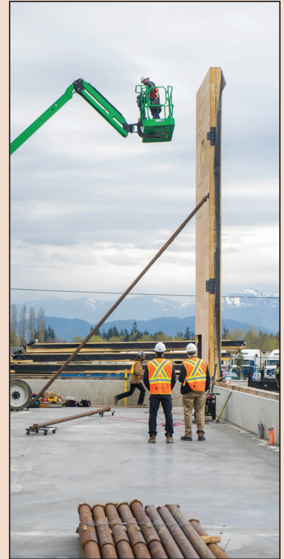
Fig. 4.6: Full-height wall panels
