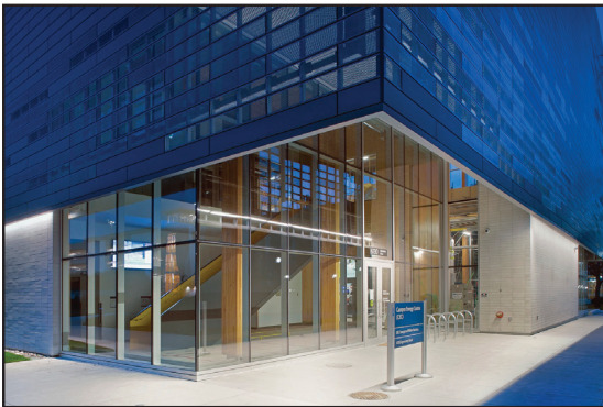
Fig. 3.7: The exterior zinc screen rises at the corner to reveal the main entrance
