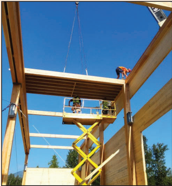
Fig. 2.10: The roof panels sit on ledgers attached to the glulam beams
