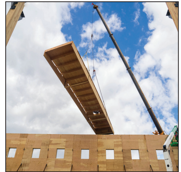
Fig. 4.4: Roof panel being lifted into place
