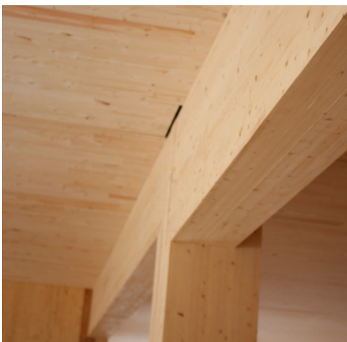
Figure 2.14. Origine, Quebec City. 13-storeys post-and-beam with CLT. (Photo: D. Moses)
