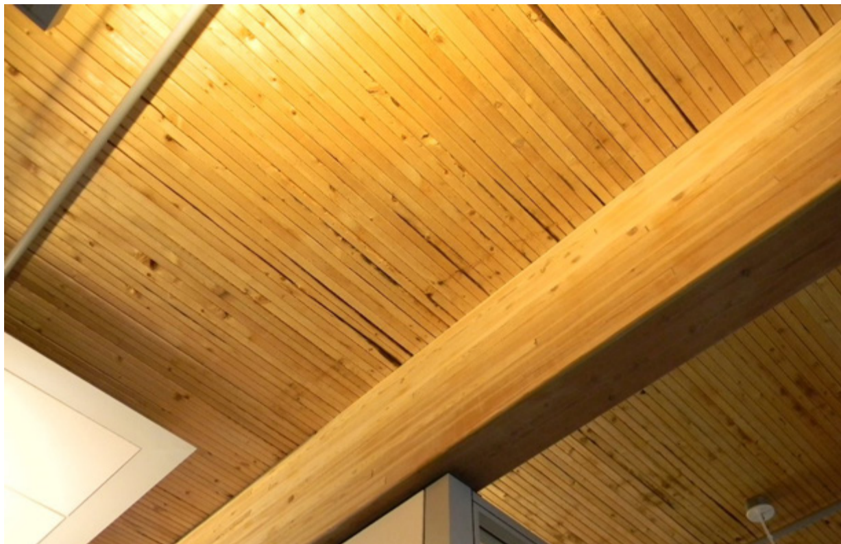
Figure 2.7 Nail-lam floor (Photo: M. Alexander)
