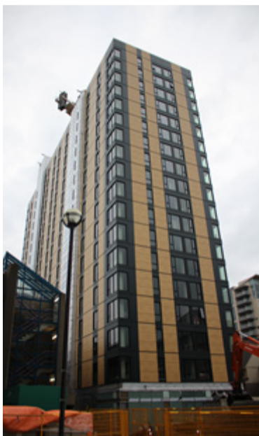
Figure 2.11. Brock Commons, UBC, Vancouver. 18-storeys. (Photo: D. Moses)
