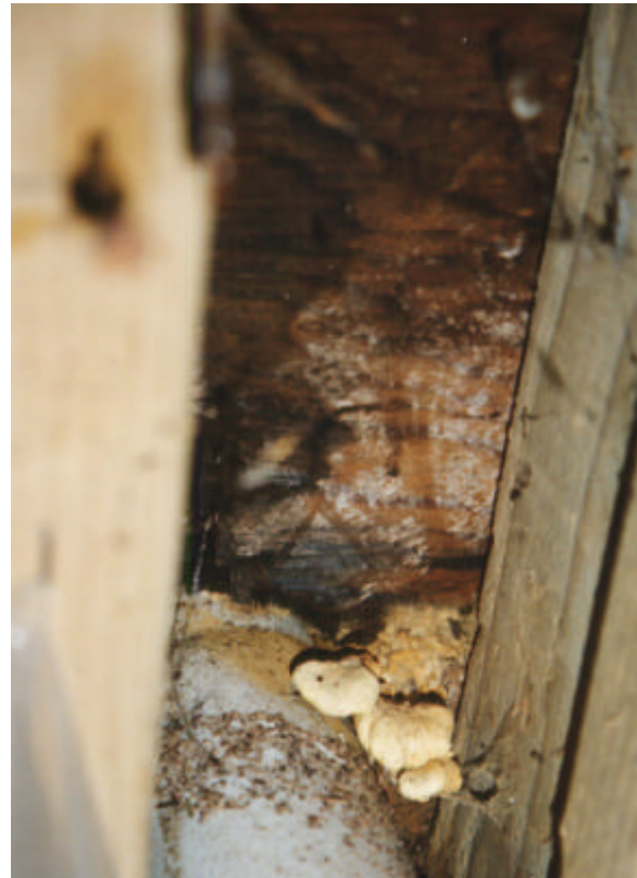
Figure 6: A fruiting structure of the brown-rot fungus Tapinella Panuoides on a Vancouver condominium
