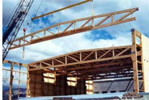
Long spans without intermediate supports create large open spaces architects and designers can use with complete freedom. Partitions can be moved without compromising the structural integrity of the building. Framing a roof with wood trusses can be accomplished in half the time required for a conventional rafter based system. In addition to flexibility and cost effectiveness trusses are used for the following reasons:
