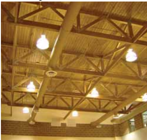
Heavy timber roof in a non-combustible building
