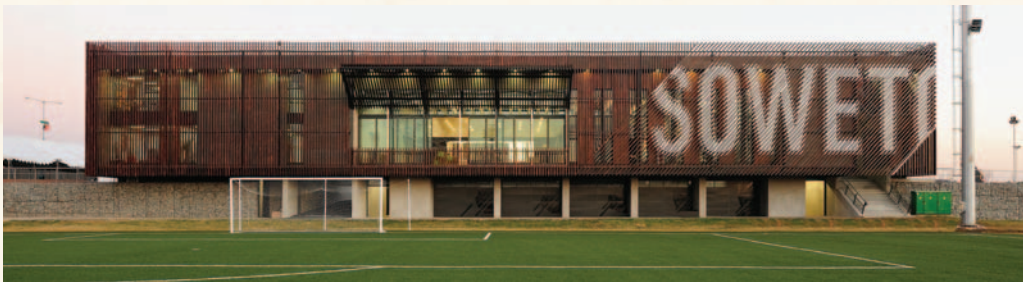
Football Training Centre, Soweto
