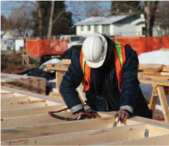
On-site fabrication of floor panels, Hillcrest Village, Fort St. John, B.C.
