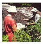
In this photo, Western Red Cedar shake roof panels are being inspected for deterioration. This site is maintained within the Malcolm Knapp Research Forest in Collaboration with the University of British Columbia Faculty of Forestry. CCA treatment not only stops decay but also reduces UV erosion by a factor of ten.
