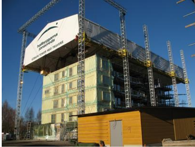
Figure 13 Using a movable tent to protect the entire construction in Sweden
