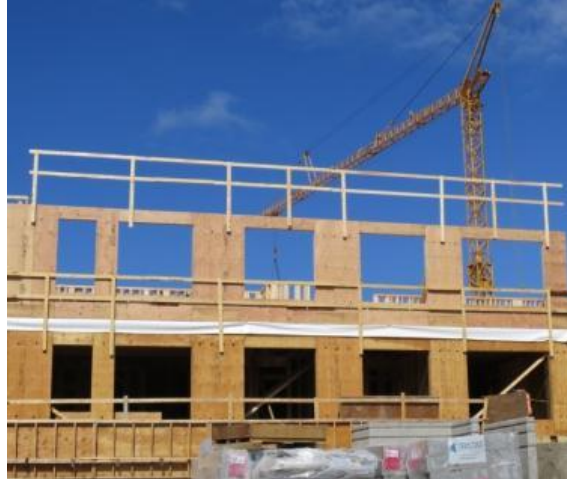
Figure 7 Using prefabricated framing for multi-unit light wood-frame construction
