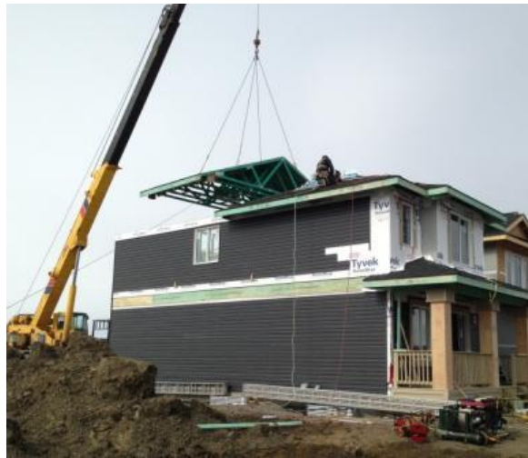
Figure 8 Installing a modular roof for a house
