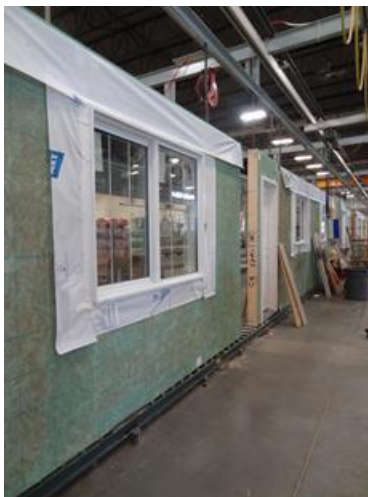
Figure 2 Prefabrication of building assemblies in a factory
