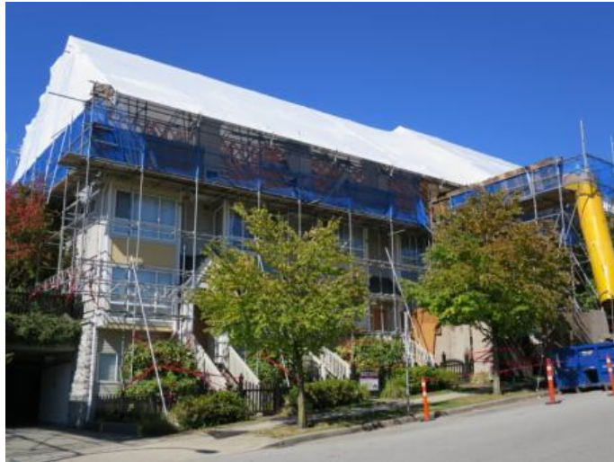
Figure 11 Weather protection during retrofit of a building in Vancouver
