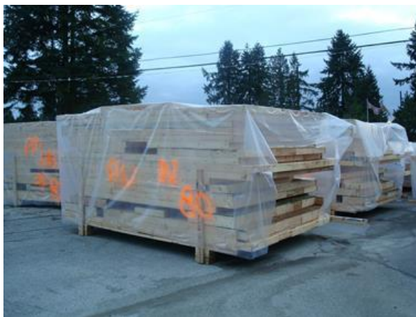
Figure 9 Covered prefabricated framing at a construction site
