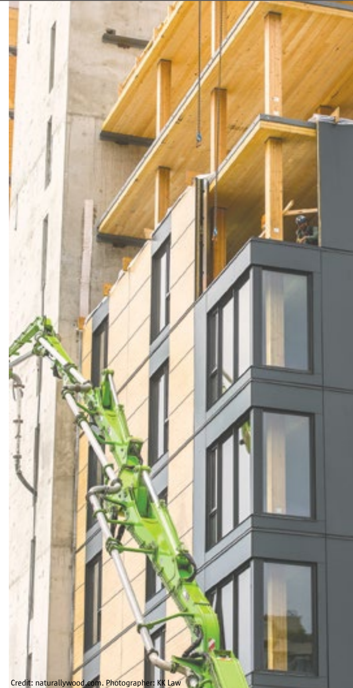
Credit: naturallywood.com. Photographer: KK Law Pumping concrete – Stairs and landings
