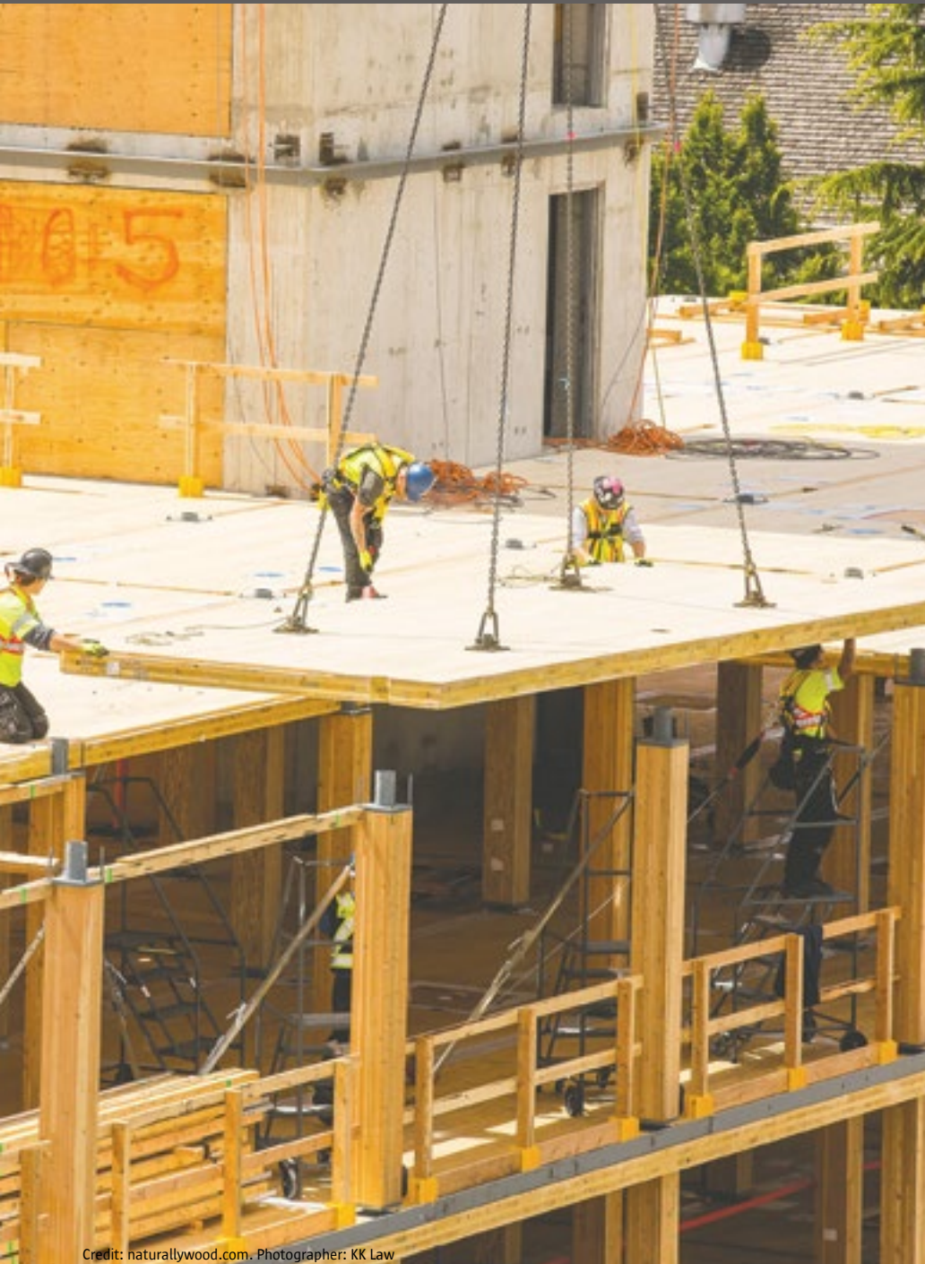
CLT panel installation
