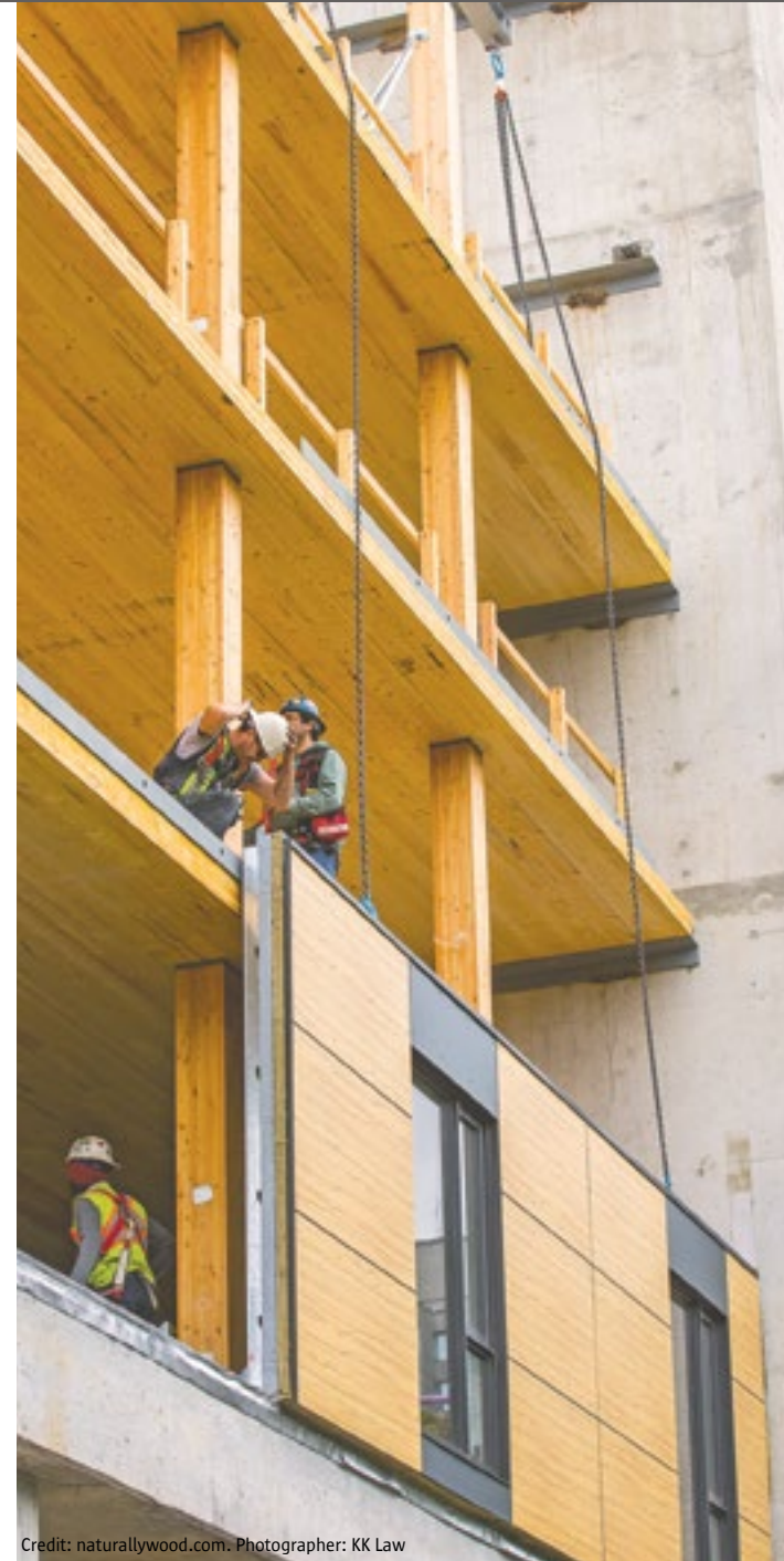
Building envelope panel installation
