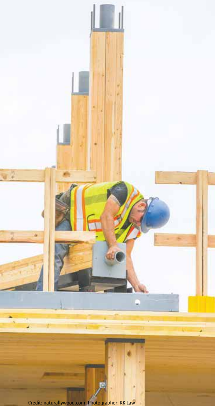
Glulam column installation
