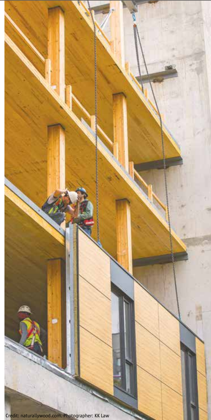
Building envelope panel installation
