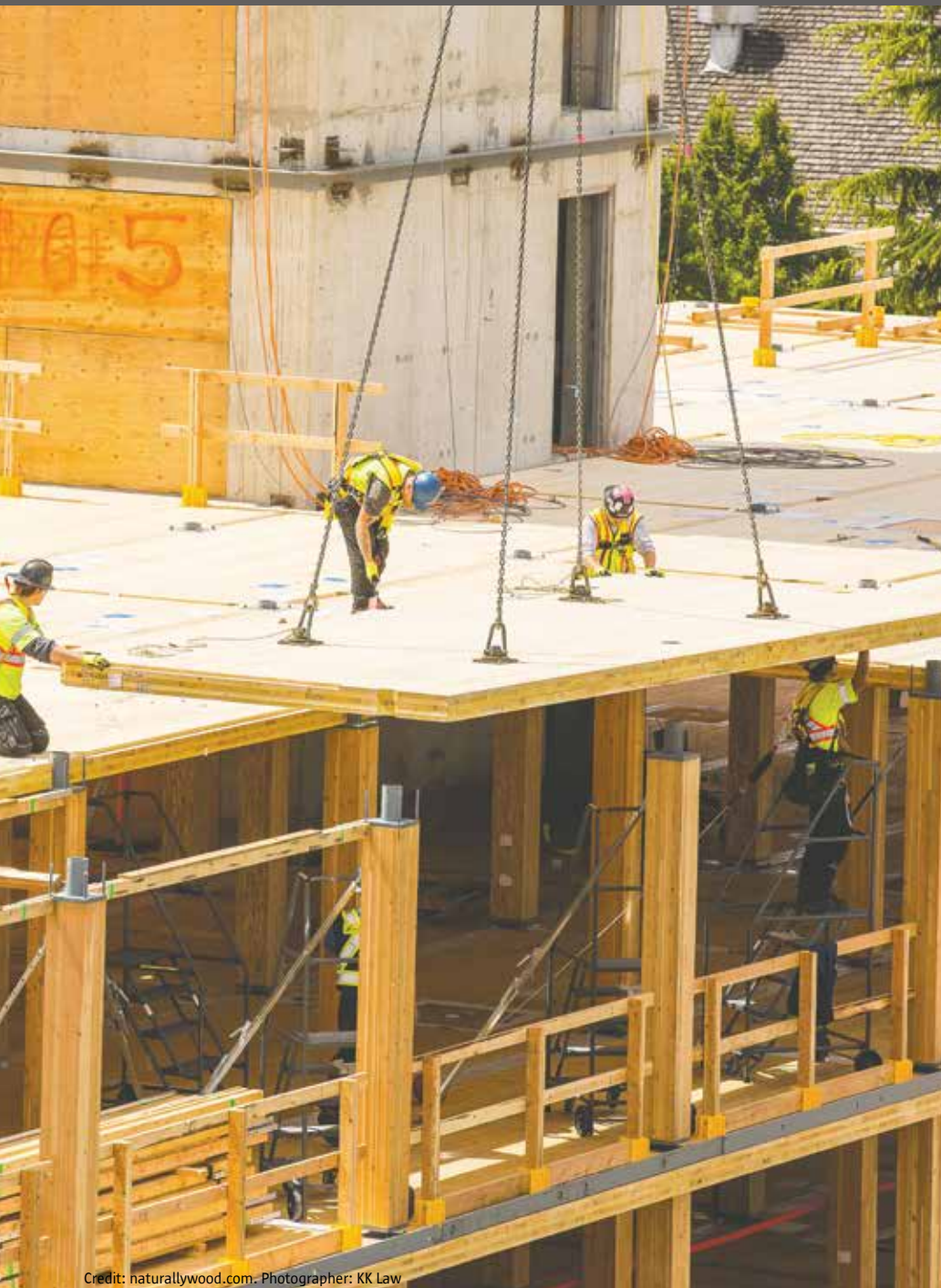
CLT panel installation
