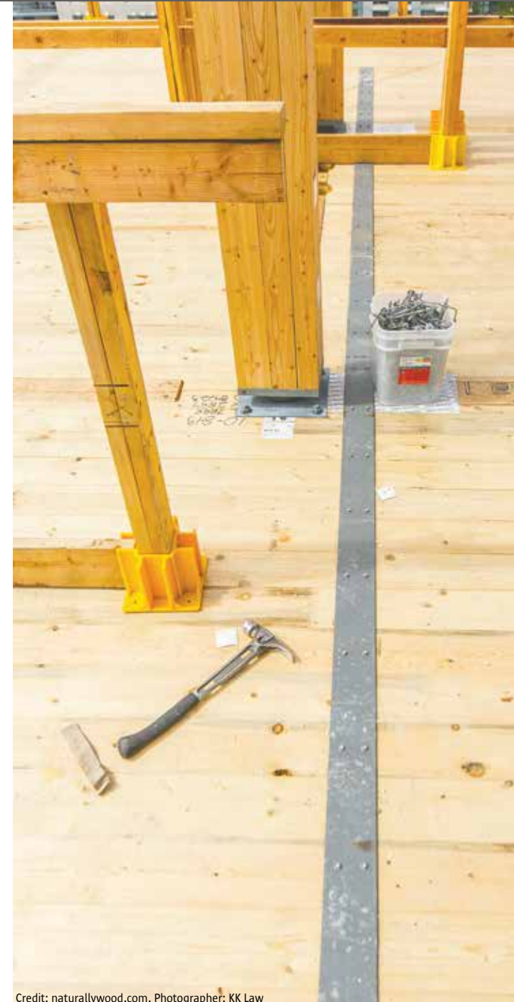
Credit: naturallywood.com. Photographer: KK Law Drag strap connecting CLT floor panels and reinforced concrete core
