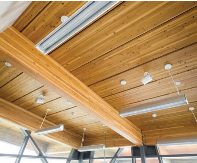
FIGURE 14 Bus Transit Station waiting room ceiling
