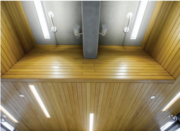
FIGURE 4 Wood ceiling in the MacEwan LRT Station waiting room
