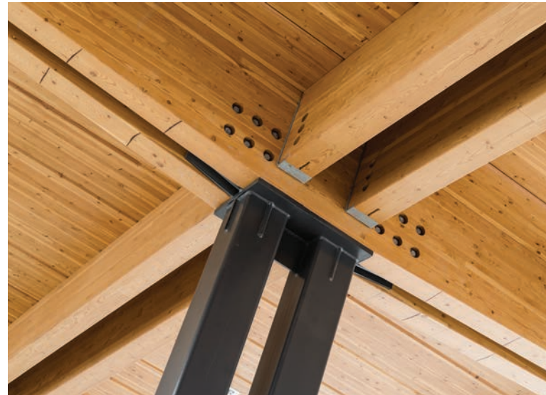
FIGURE 6 Concealed connections
