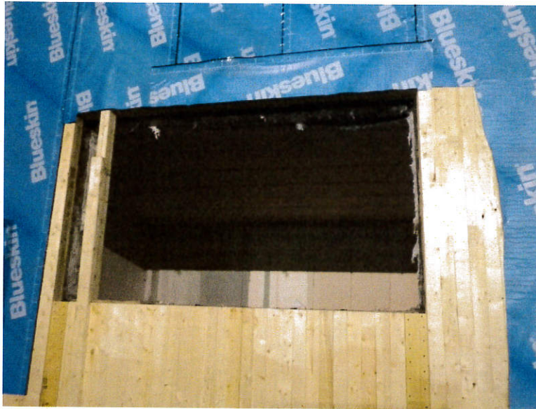
Figure 4. Wall system under construction.
