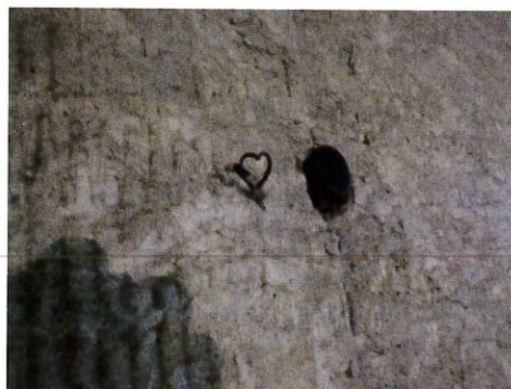
Tension mounted TC and heat-flux transducer
