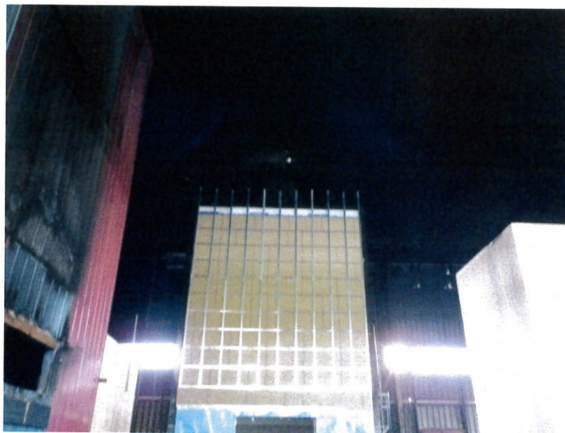
Figure 5. Installation of Roxul insulation.
