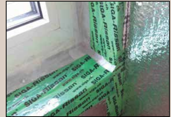
Fig. 2.10: Taping of vapour barrier at window
