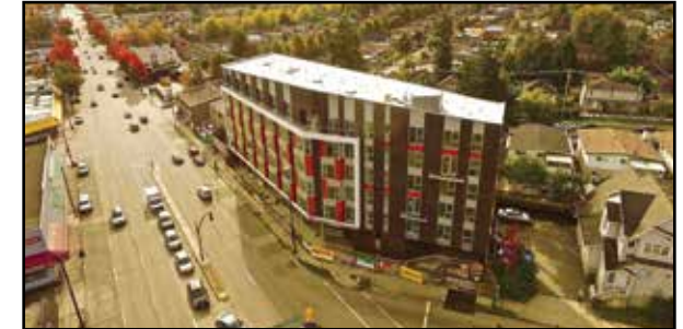
Fig. 3.2: Aerial photo showing urban context
