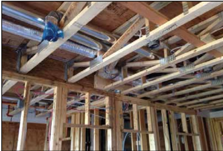
Fig. 3.10: Parallel chord trusses enable services to be run within the depth of the floor
