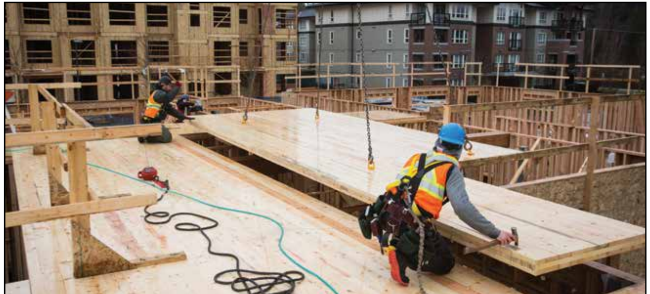
Fig. 4.4: Installation of CLT panels
