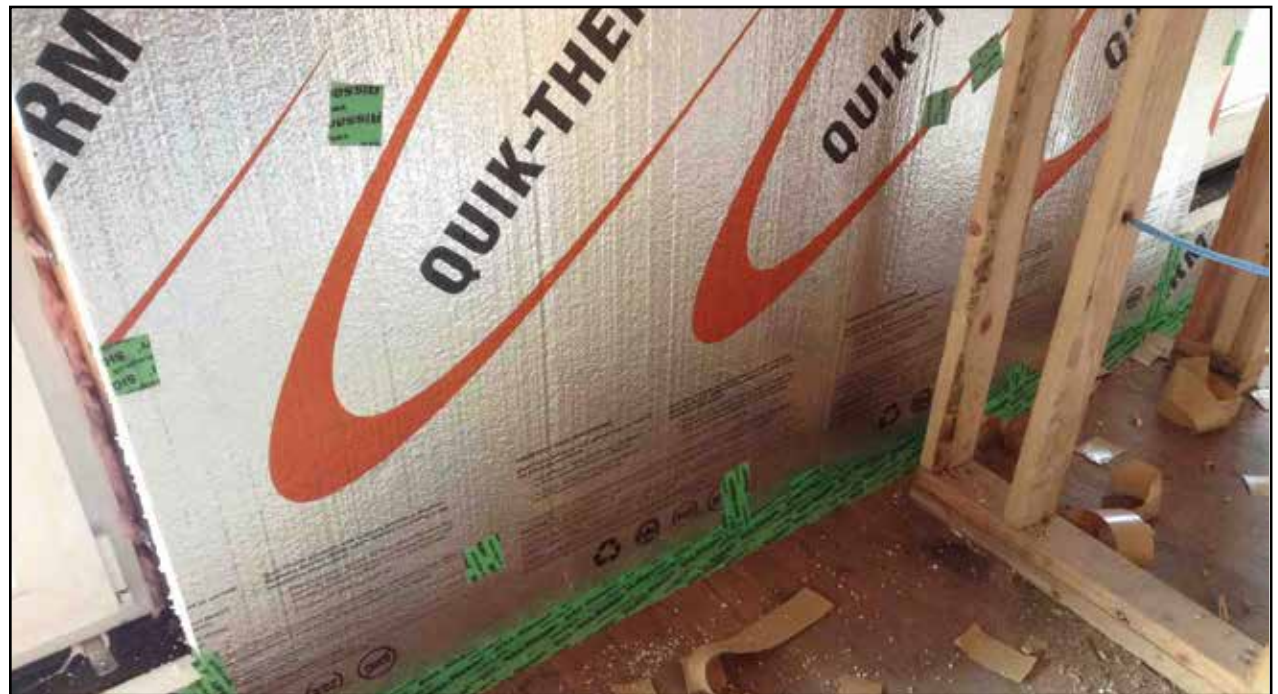
Fig. 2.3: Installation of rigid air barrier
