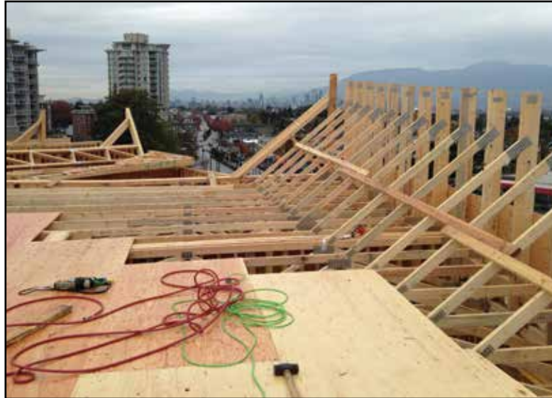
Fig. 3.9: Construction of roof
