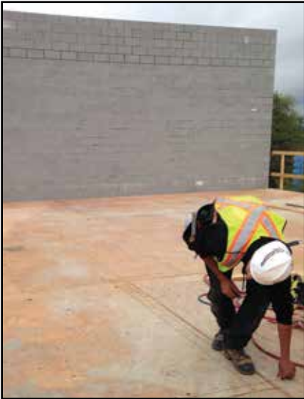
Fig. 3.7: Concrete masonry fire-resistance-rated wall
