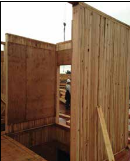
Fig. 3.8: Installation of NLT elevator shaft
