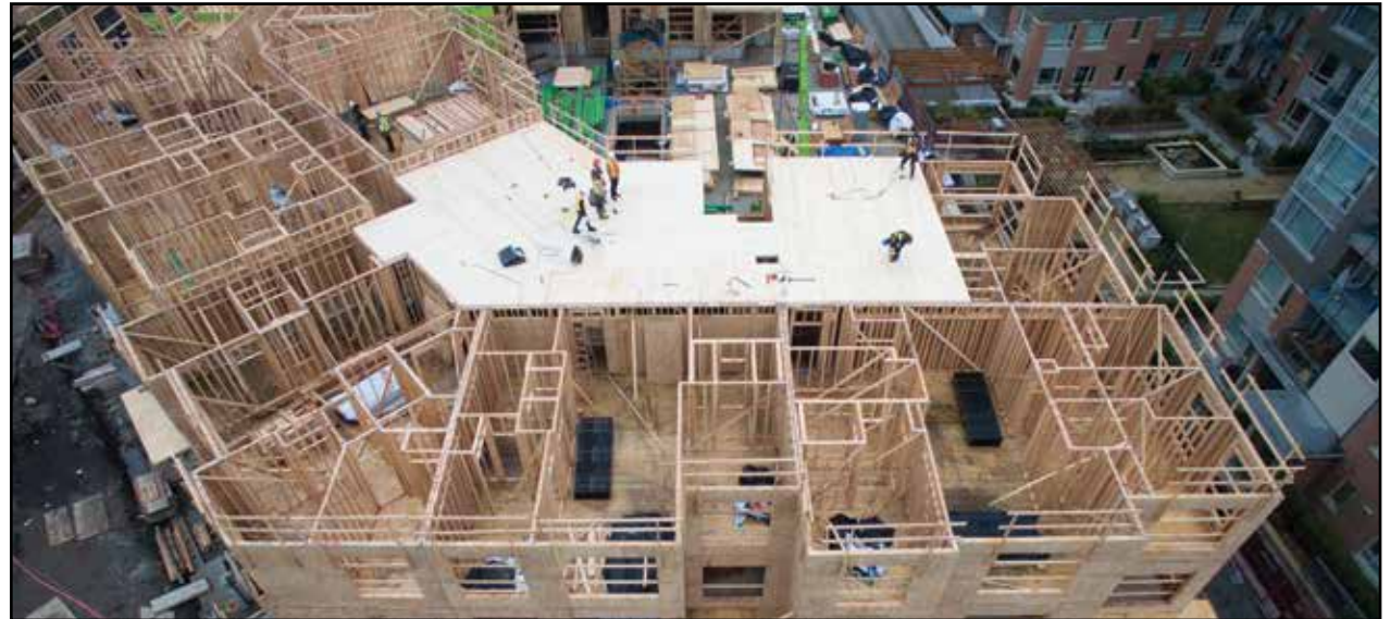
Fig. 4.11: Aerial view of CLT floor being installed
