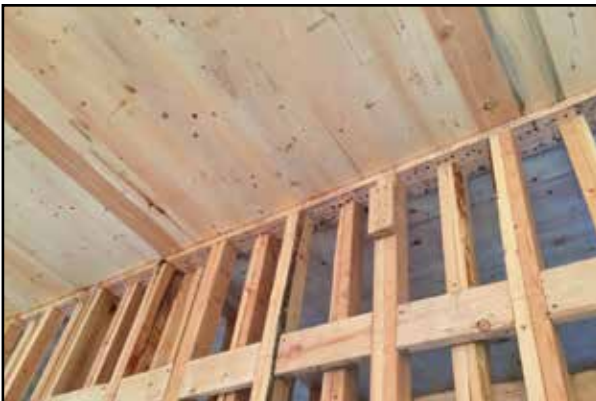
Fig. 4.2: Light wood frame walls support CLT floors
