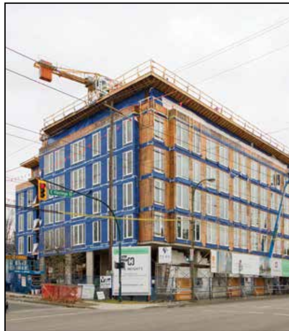
Fig. 2.5: View showing vapour barrier wrapped over floor lines
