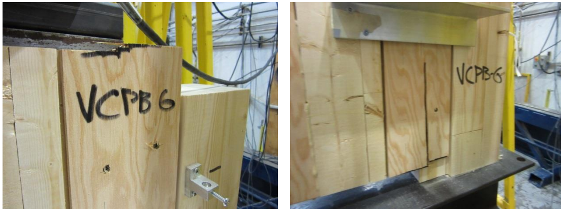
Figure 9. Shear through the plywood thickness observed for specimen VCPB 6
