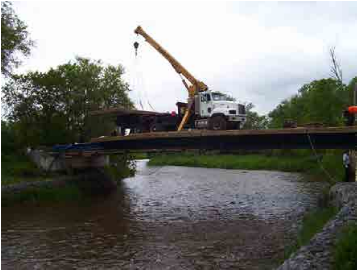
Photo Credit: Guardian Bridge Rapid Construction Inc.
