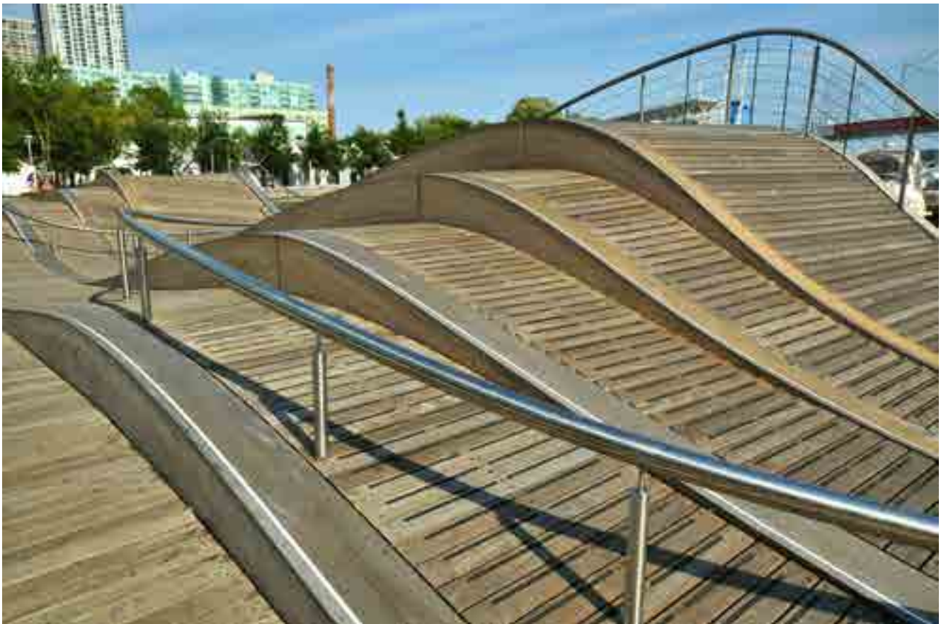
Figure 1.4.3. Waterfront wave decks, Toronto. Yellow cedar glulam timber girders. Photo provided courtesy of the Ontario Wood WORKS! Wood Design Awards program.
