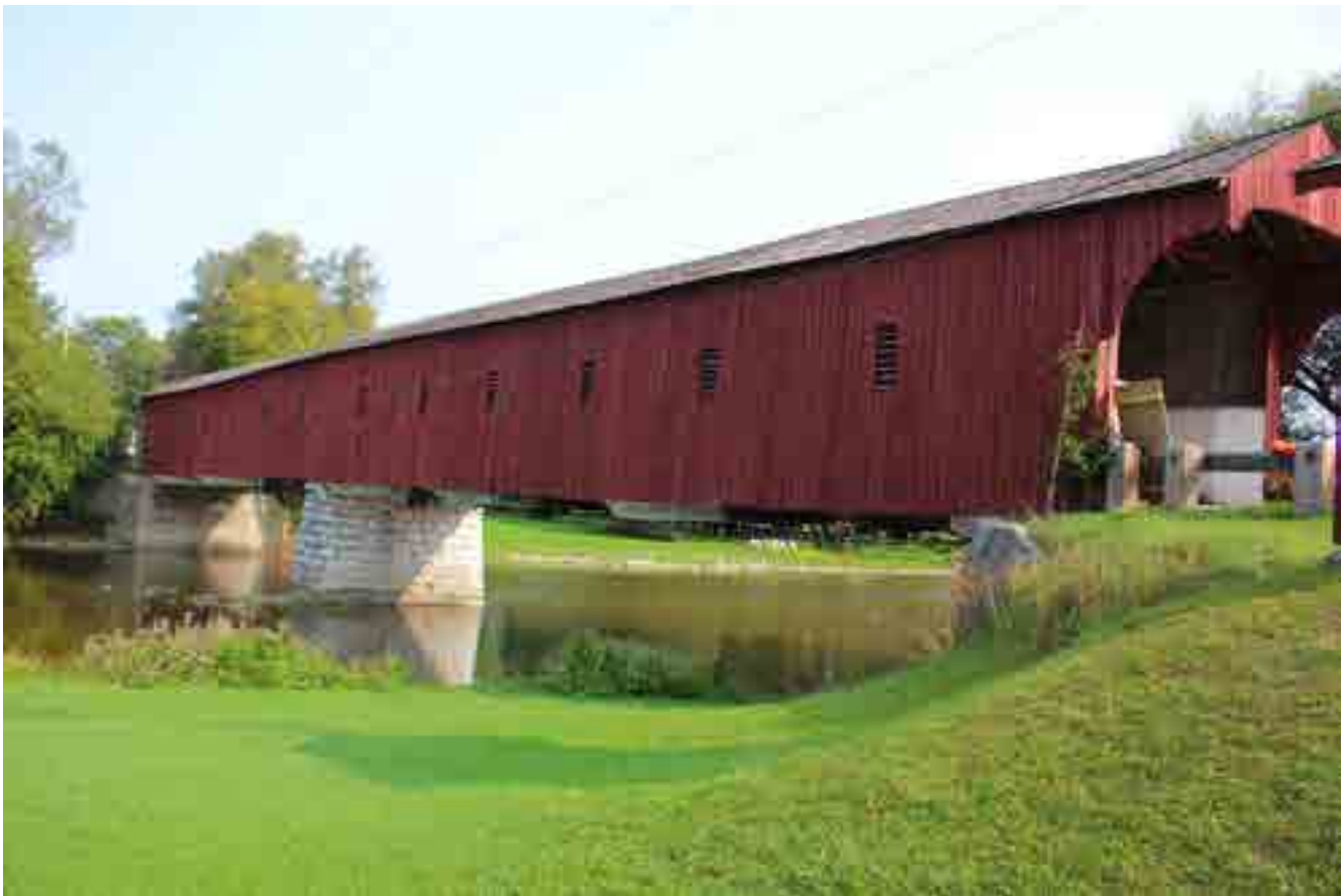
West Montrose Bridge, Ontario, D. Moses
