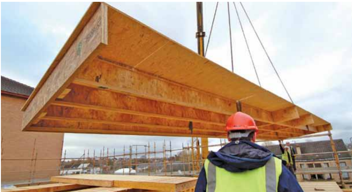
5-Storey Apartment Block Pre-fabricated floor system installation
