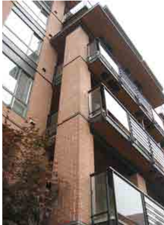
FIGURE 6.5 – THE SHORE: BALCONY SUPPORTS CLAD IN MASONRY
