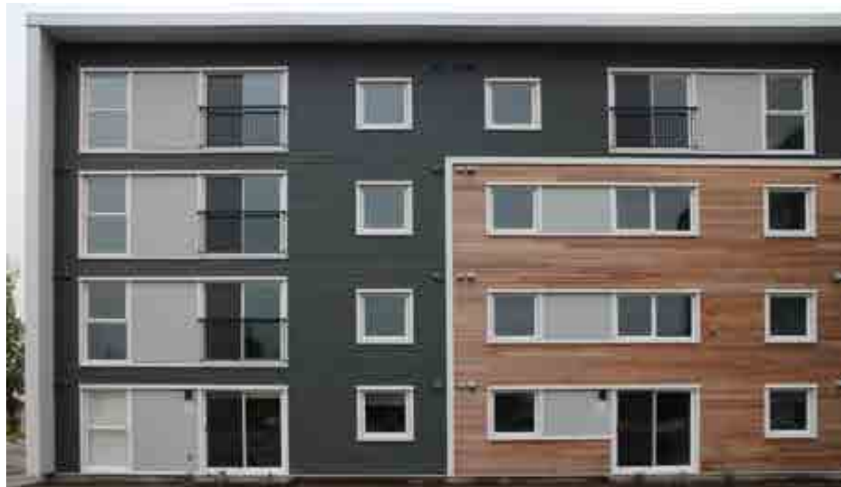
FIGURE 3.1 – HILLCREST VILLAGE: A COMBINATION OF FIBRE CEMENT PANELS AND CEDAR SIDING IS USED TO MINIMIZE WEIGHT
