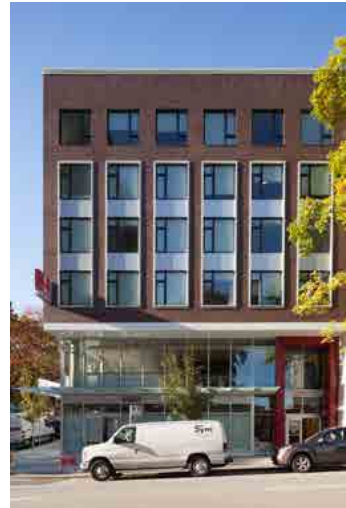
FIGURE 3.2 – SFU DOWNTOWN RESIDENCE: THE FULL-WIDTH BRICK CLADDING EXTENDS FROM THE THIRD TO THE SIXTH FLOOR
