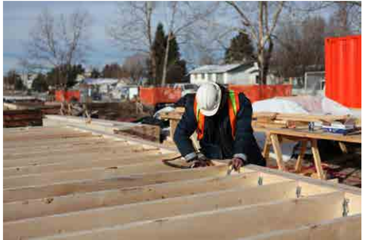
FIGURE 7.2 – HILLCREST VILLAGE: SITE PREFABRICATION OF FLOOR PANELS
