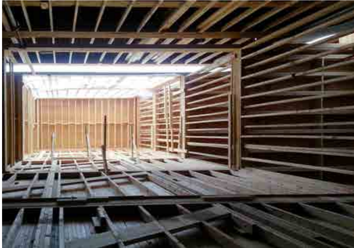
FIGURE 5.3 – HILLCREST VILLAGE: AS IS TYPICAL IN MID-RISE CONSTRUCTION, STAIR WELLS ARE CONSTRUCTED WITH LIGHT WOOD-FRAME ELEMENTS
