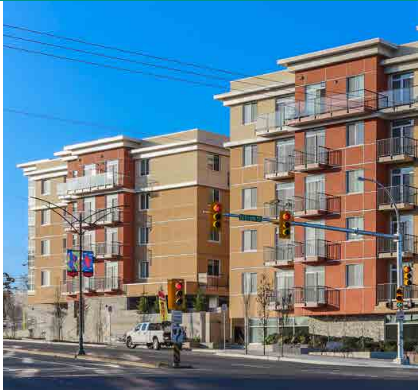
FIGURE 2.4 – HERONS LANDING, TOGETHER WITH THE ARDEA, IS THE FIRST RENTAL HOUSING PROJECT TO BE BUILT IN SAANICH IN 25 YEARS
