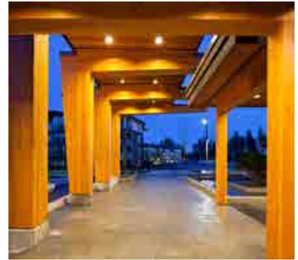
FIGURE 5.1 – SAIL: EXTERIOR WOOD STRUCTURES SUCH AS ENTRANCE CANOPIES, MUST BE OF HEAVY TIMBER CONSTRUCTION
