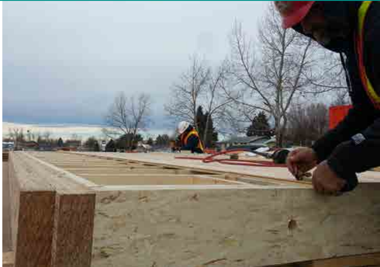
FIGURE 4.2 – HILLCREST VILLAGE: ON-SITE PREFABRICATION OF FLOOR PANELS
