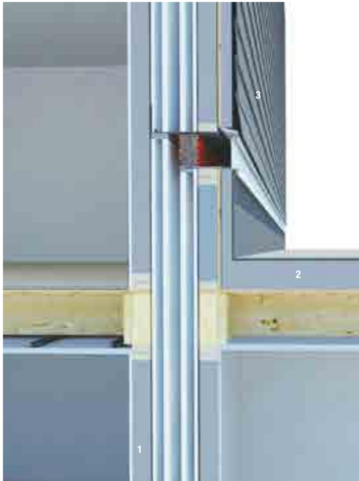
1. proprietary firewall 2. roof of four-storey building 3. exterior wall of six-storey building
