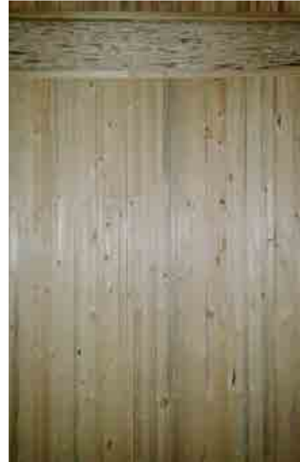
FIGURE 4.5 – HILLCREST VILLAGE: CLOSE UP VIEW OF NLT ELEVATOR SHAFT
