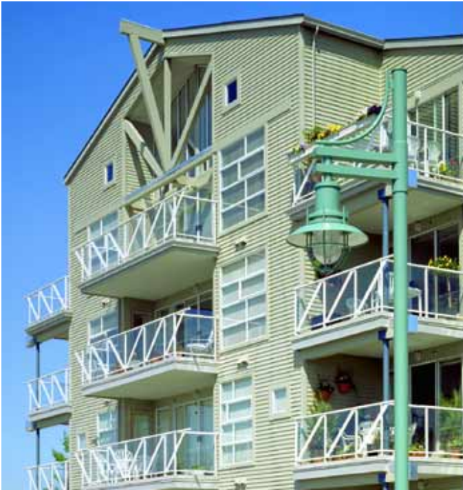
Figure 2 Four Storey Wood Frame Residential Construction
