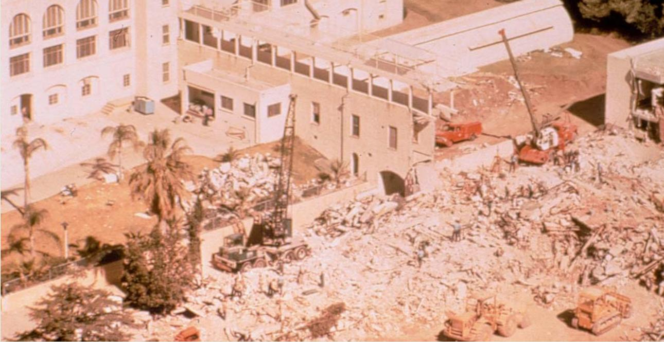
Aerial view of the damage to the San Fernando Veterans Administration Hospital and complex. The collapsed masonry structure was built in 1926, before earthquake building codes were in effect. Forty-seven deaths occurred as a result of the collapse of the structure.
