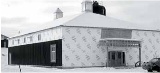
PHOTO 4: Weather-resistant barriers, used together with flashing around windows and door openings, help to keep buildings dry.
