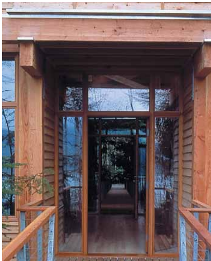
PHOTO 8: Overhangs protect end-grain of beams from moisture.
