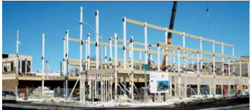
Photo: DSSAB Construction
