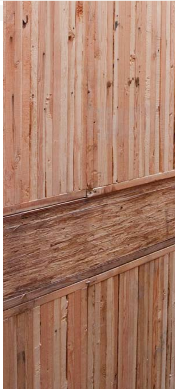
ELEVATOR SHAFT SOLID WALL FRAMING
