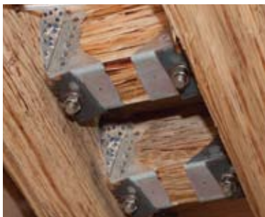
FRAMING AND CONNECTION DETAIL
