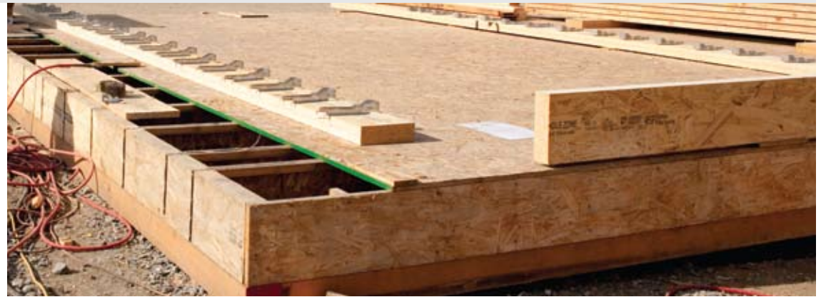
ON-SITE FLOOR PANEL PREFABRICATION
