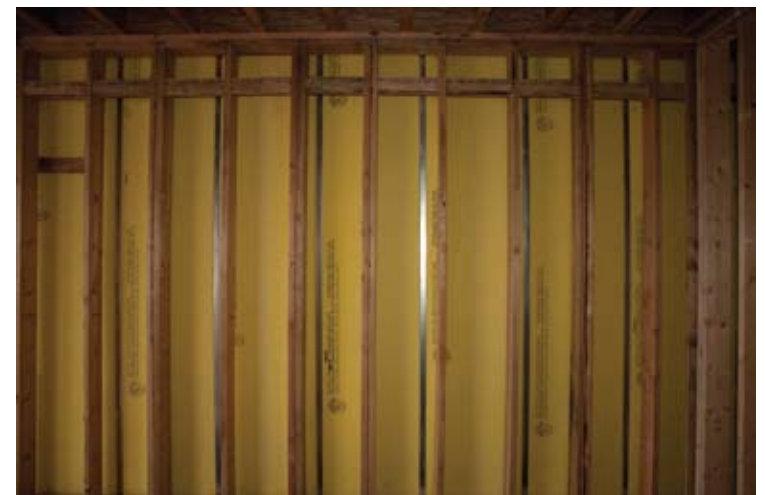
TWO-HOUR GYPSUM FIRE-RESISTANCE-RATED FIREWALL SYSTEM
