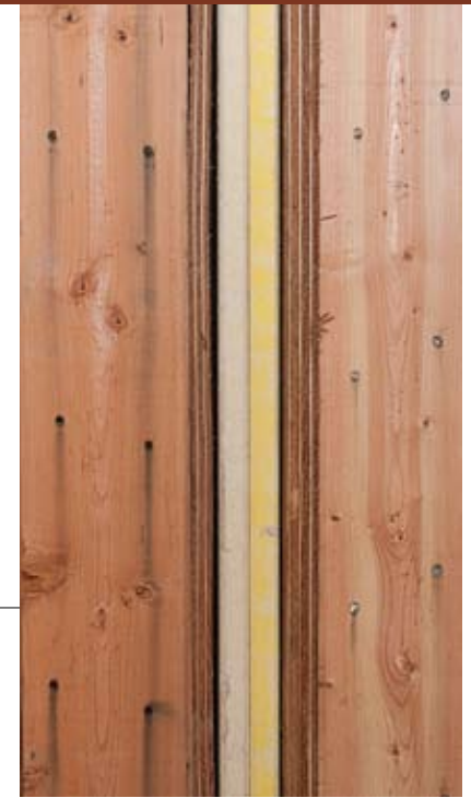
GYPSUM FIREWALL SYSTEM - A TWO-HOUR FIRE RESISTANCE RATING
