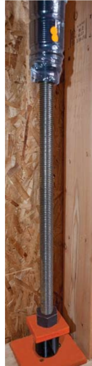
SELF-ADJUSTING TIE-ROD SYSTEM - SIMPSON STRONG-TIE® ANCHOR TIEDOWN SYSTEM (ATS)
