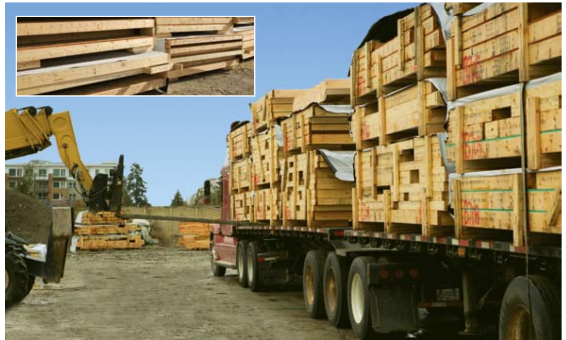
OFF-SITE WALL PANEL PREFABRICATION
