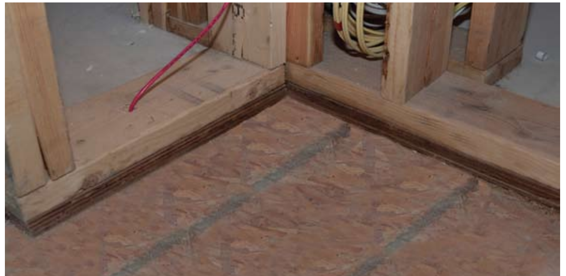
ONE-INCH-THICK GYPSUM-CONCRETE TOPPING / ONE-INCH PLYWOOD BOTTOM PLATE
