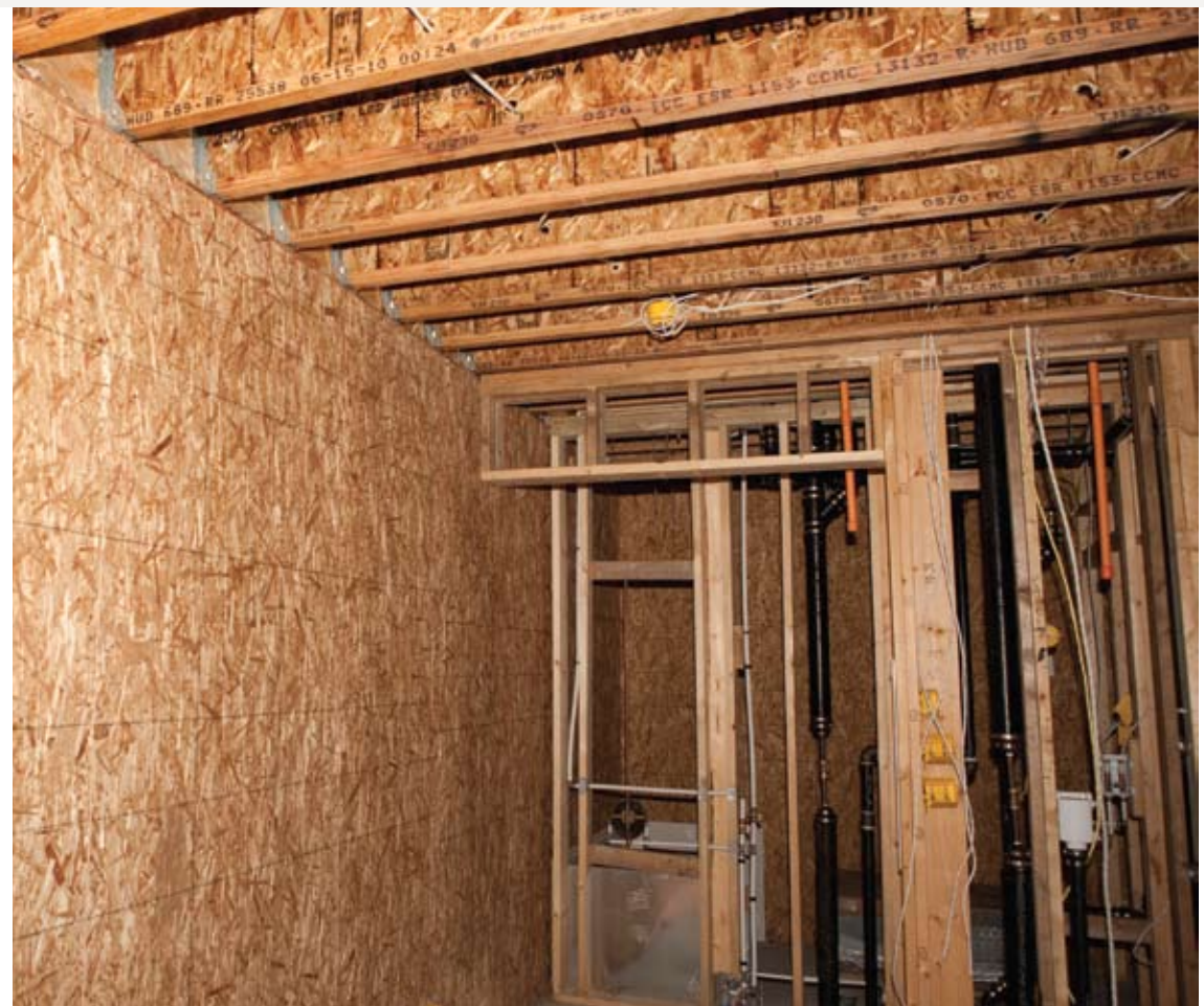
ORIENTED-STRAND-BOARD (OSB) SHEATHED SHEARWALL
