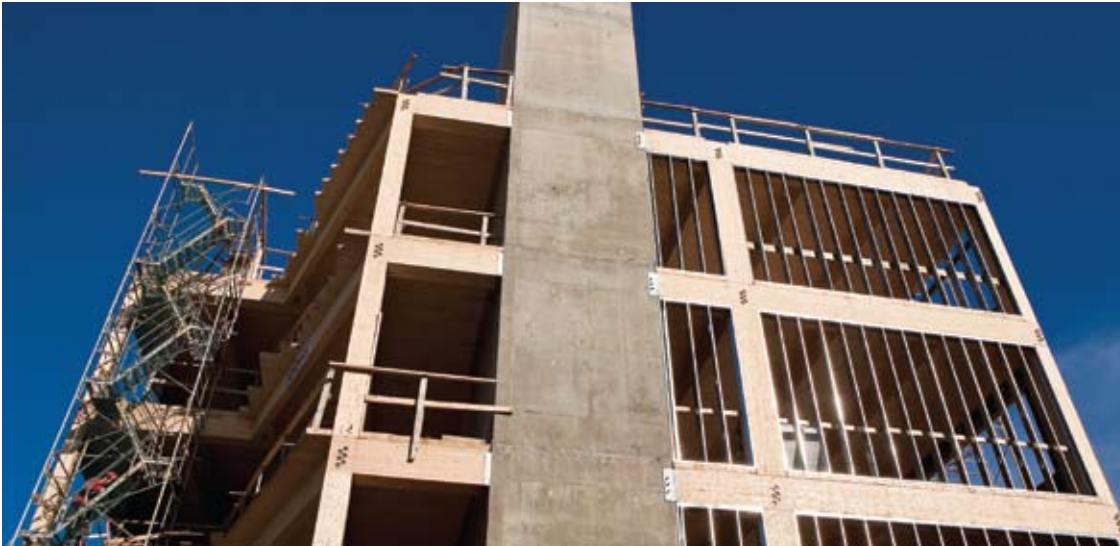
HYBRID CONSTRUCTION: QUÉBEC - FONDATION PROJECT (PHOTO COURTESY OF CECOBOIS)
