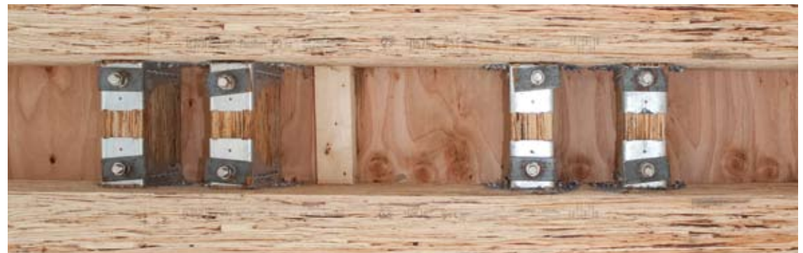
FRAMING AND CONNECTION DETAIL
