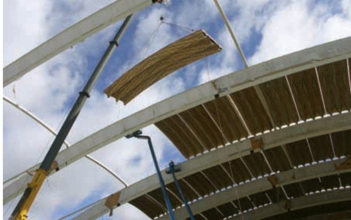
Placing a WoodWave panel
