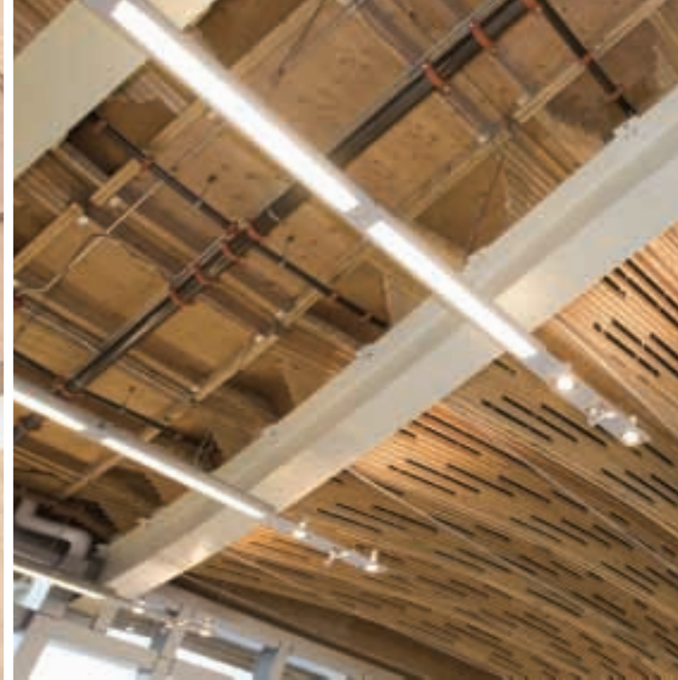
Sprinkler system connections and pattern
