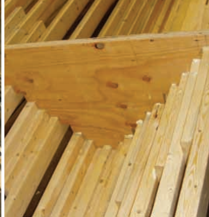
Panel Vee with plywood gusset positioned and glued
