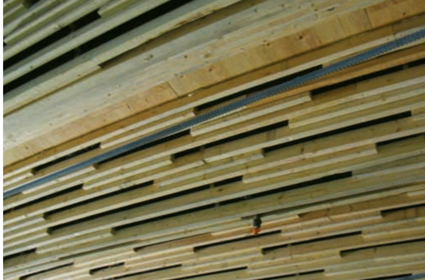
Panel Vees – underside
