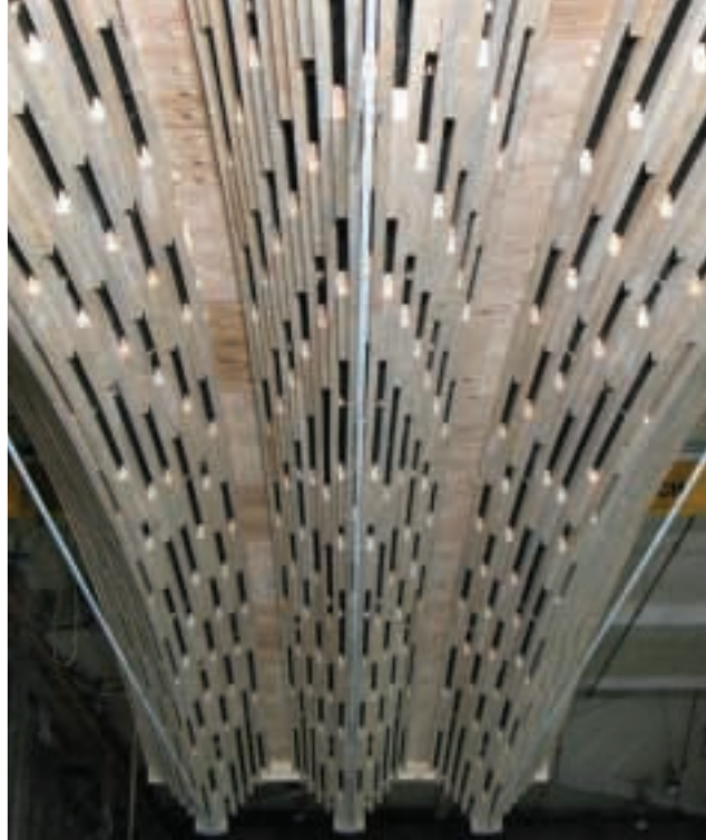
Panel Vees – strand orientation and spacing
