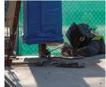
Placement of column for welding to the baseplate
