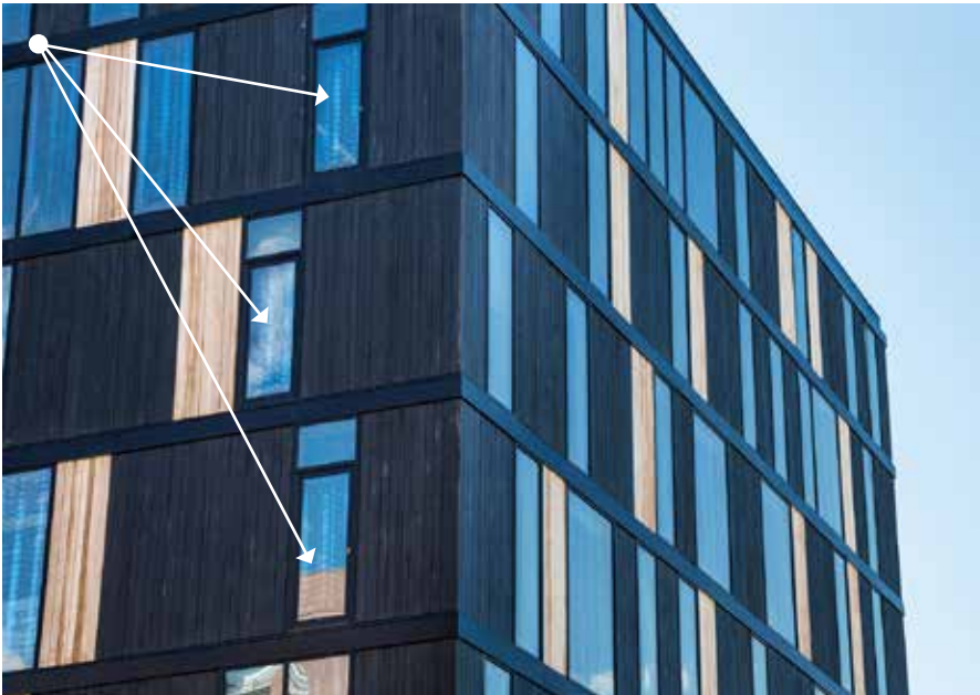
One of the two tiers of fire access doors integrated into the George Street façade
