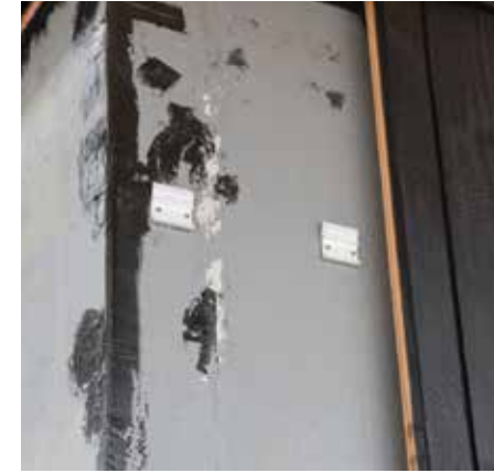
Mounting clip on SIP panel for mounting the cladding panel
