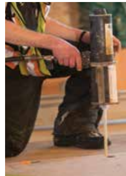
Epoxy injection for securing the HSK plate
