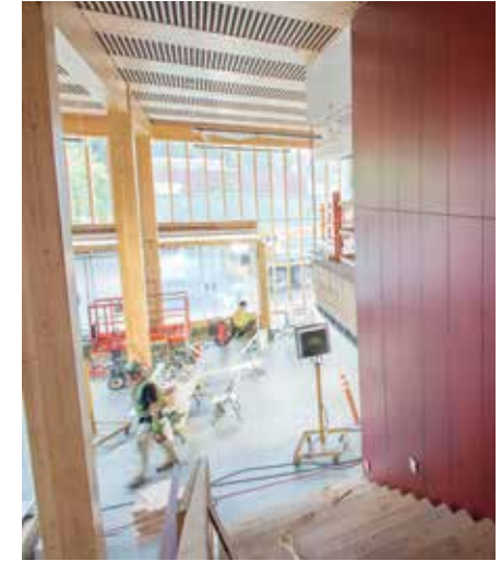
Red-stained plywood feature wall during construction
