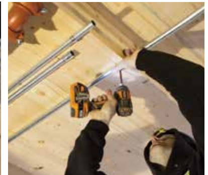
Installation of services below CLT floor
