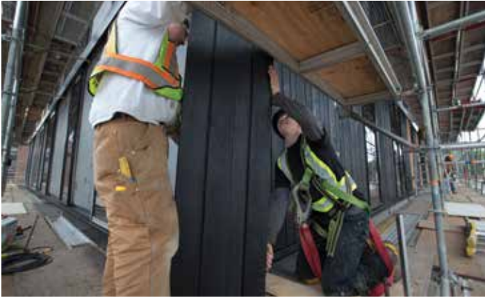
Installation of a cladding panel with charred siding
