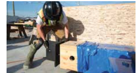
Installation of glulam column-to-column connector
