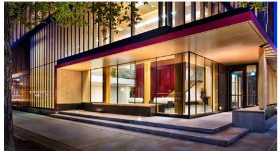
View of entrance
