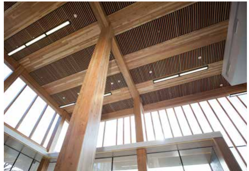
Underside of mezzanine
