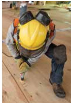
Saw kerf (left of the worker) ready for HSK plate insertion
