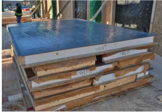
SIP panels with air barrier membrane on the exterior face
