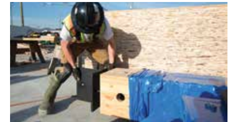
Installation of glulam column-to-column connector
