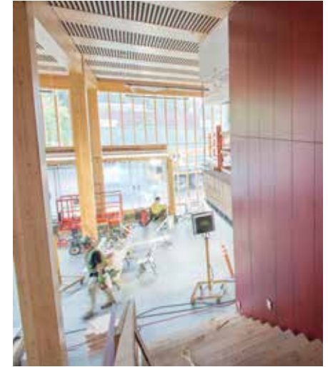
Red-stained plywood feature wall during construction
