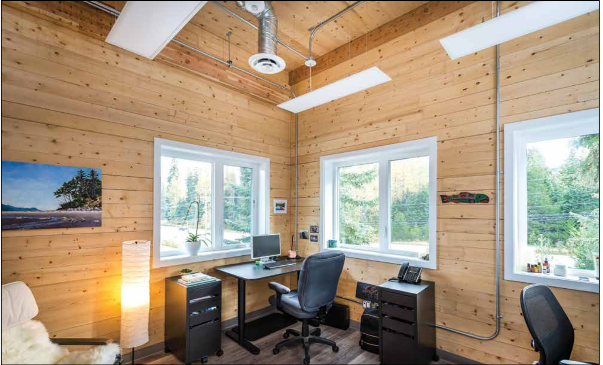
3.19 Interior of finished building showing exposed CLT panels (Andrew Dalton Photography, Courtesy AKA architecture + design)
