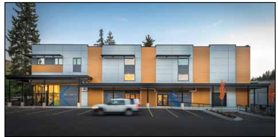
3.3 North elevation: wood building showing pattern of joints in cladding (AKA architecture + design)
