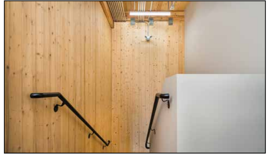
3.4 CLT panels left exposed as an interior finish (Andrew Doran Photography, Courtesy AKA architecture + design)
