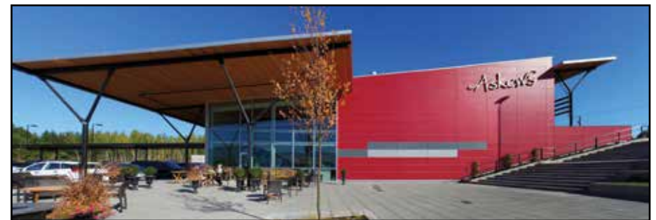
2.5 West elevation, canopy and stairs to street (Florian Maurer)
