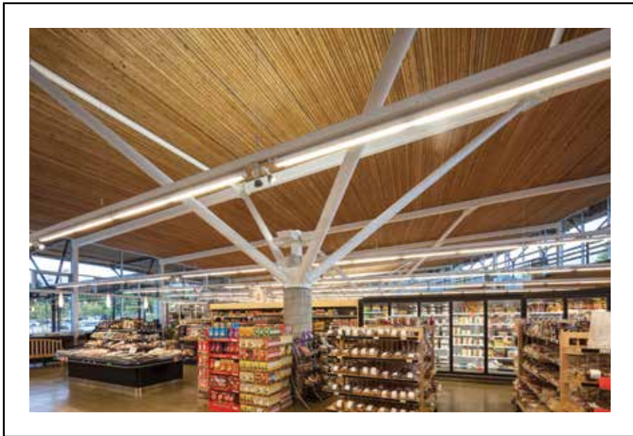
2.7 View of tubular steel tree column (Derek Lepper Photography, Courtesy Allen+Maurer Architects Ltd.)
