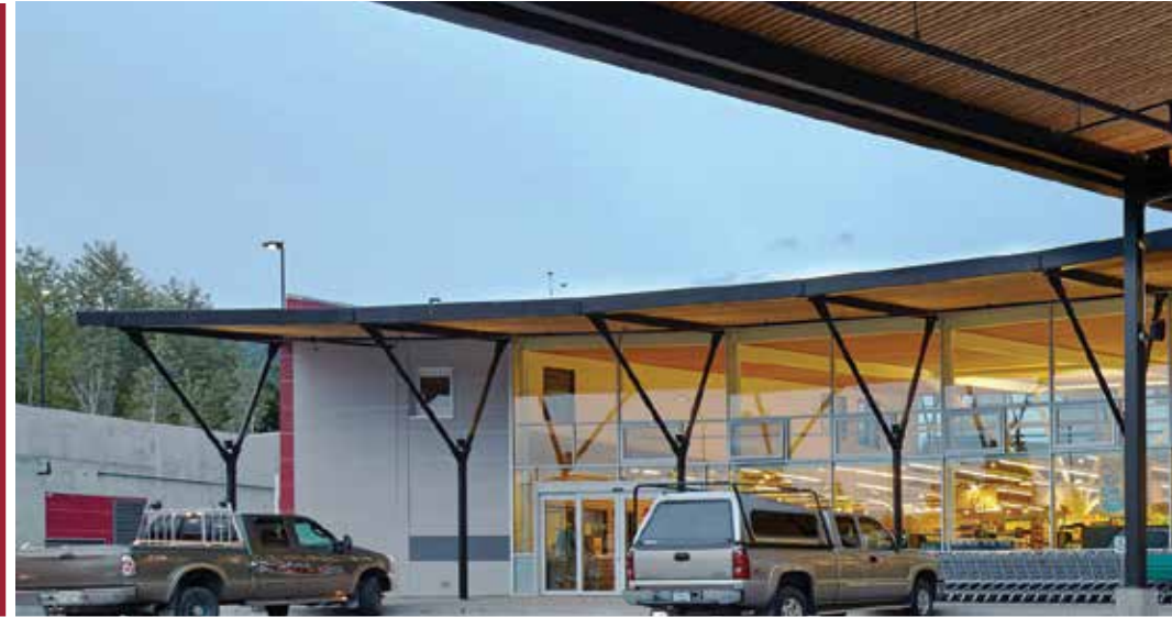
1.1 Askew’s Uptown Supermarket (Martin Knowles, Courtesy Allen+Maurer Architects Ltd.)
