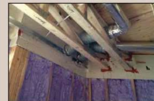
Fig. 3.5: The edges of the drywall were caulked to meet fire and acoustic requirements
