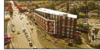
Fig. 3.2: Aerial photo showing urban context
