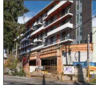
Fig. 3.3: Restricted site access at rear of property
