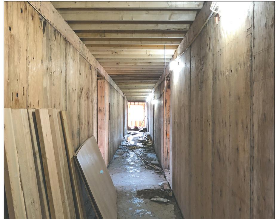
2.11 Post-disaster framing includes many laminated post and shear walls with plywood on both sides.
