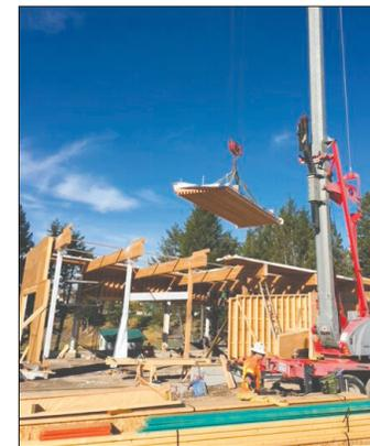
3.12 DLT panels were lifted into place by crane.
