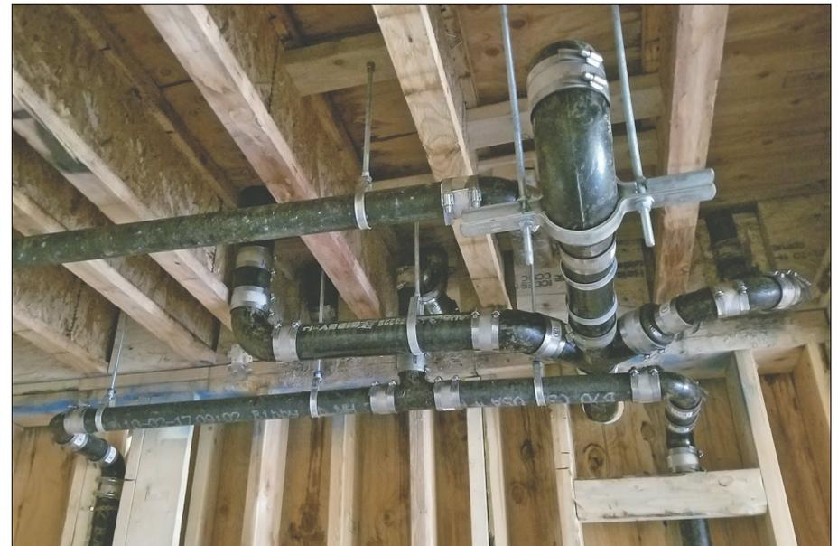
2.12 The overall height restriction required careful routing of mechanical services through the wood floor structure.
