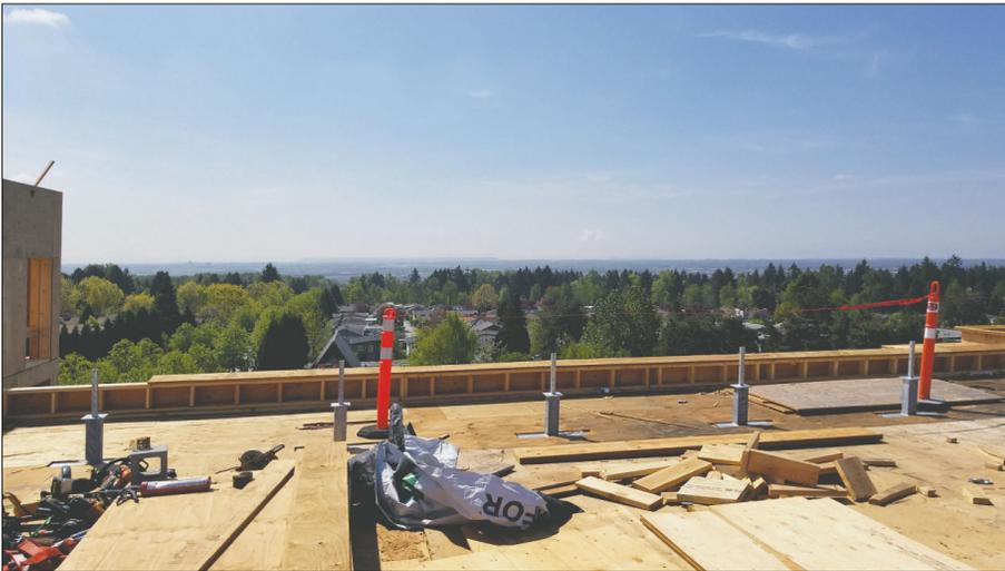
2.13 Roof construction showing line of steel stanchions required to support fence posts for play area.
