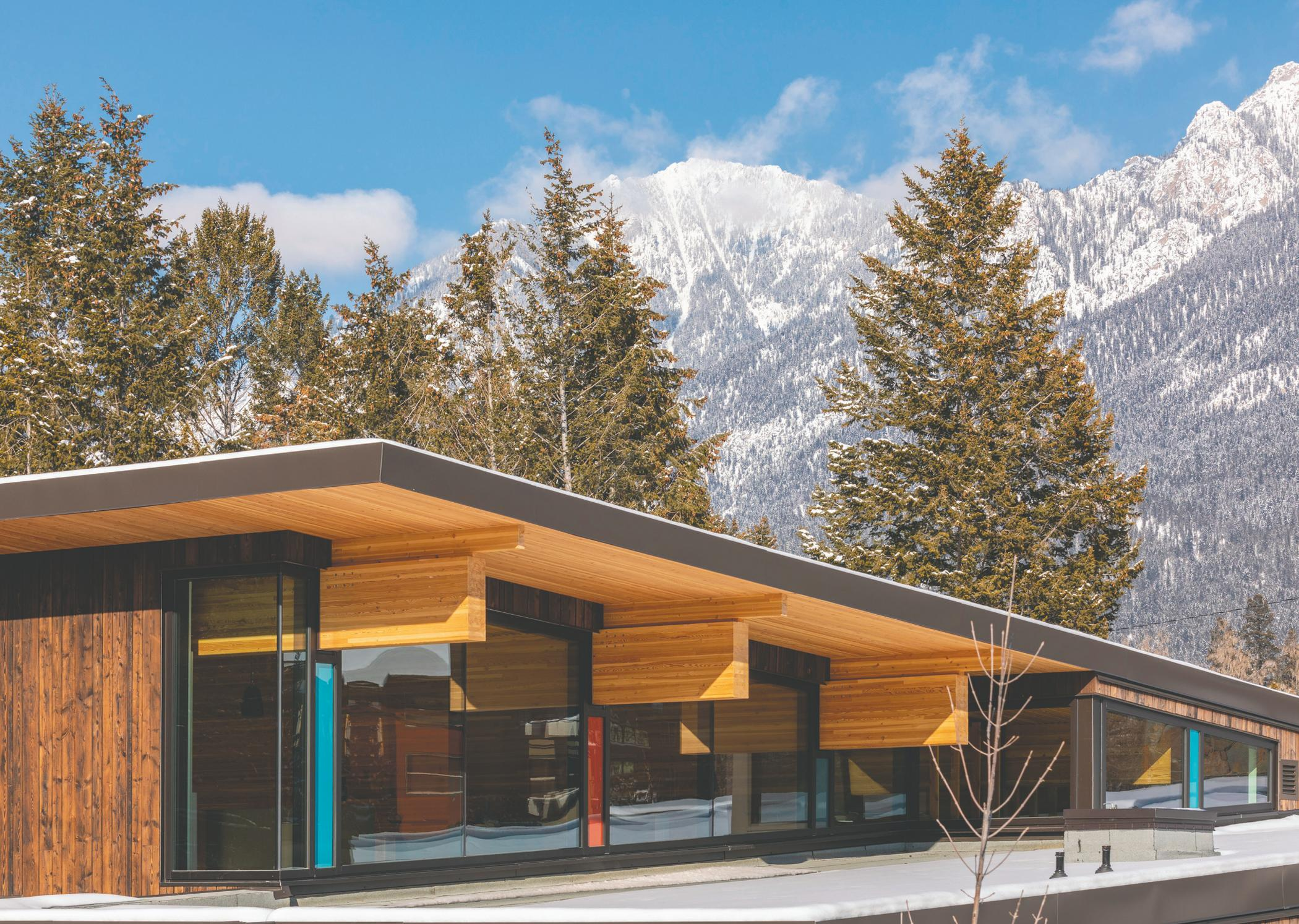
3.2 The building incorporates 288 cubic metres of locally harvested wood, milled or fabricated into a wide variety of products.
