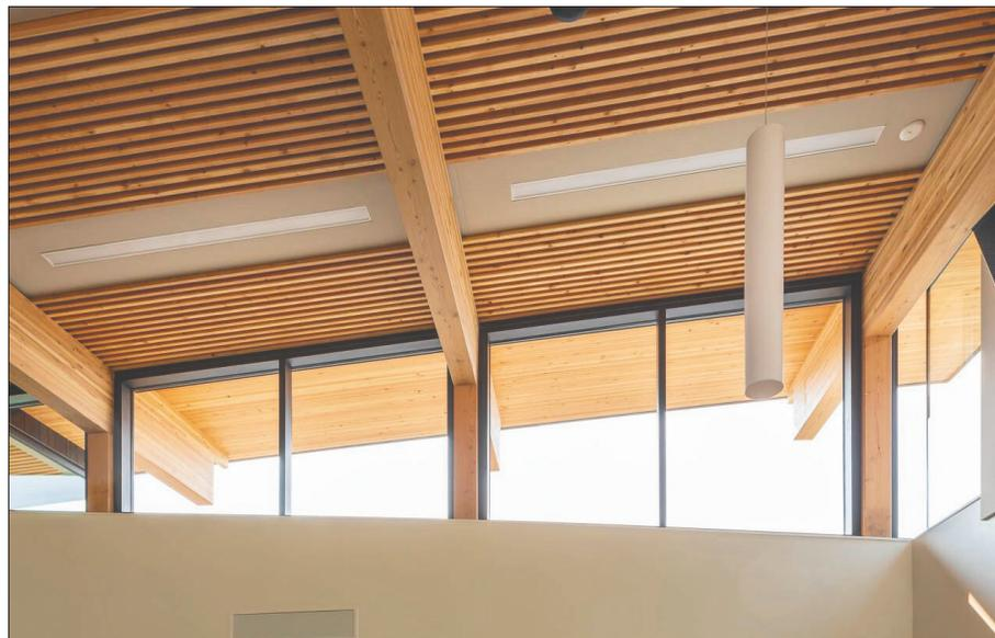
3.11 DLT panels have alternate 2x4 and 2x6 members creating a corrugated soffit. The 600 mm gap between panels accommodates lighting and is concealed with an acoustic panel.
