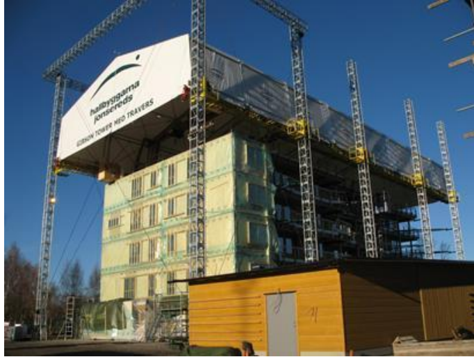
Figure 8 Using a liftable temporary roof to protect timber construction in Sweden.
