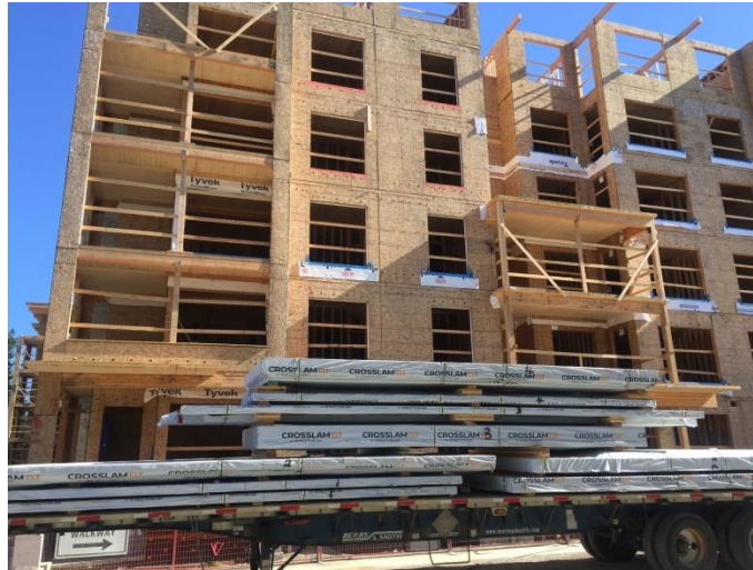
Figure 8 Wrapped CLT panels before installation.
