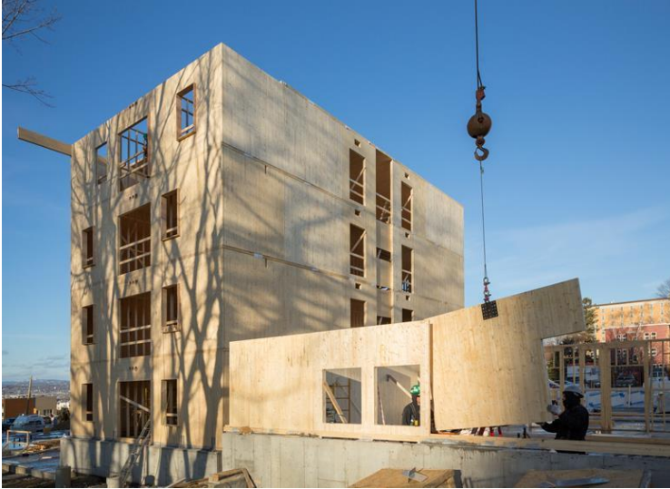
Figure 7 Installation of pre-cut CLT in a project in Quebec.
