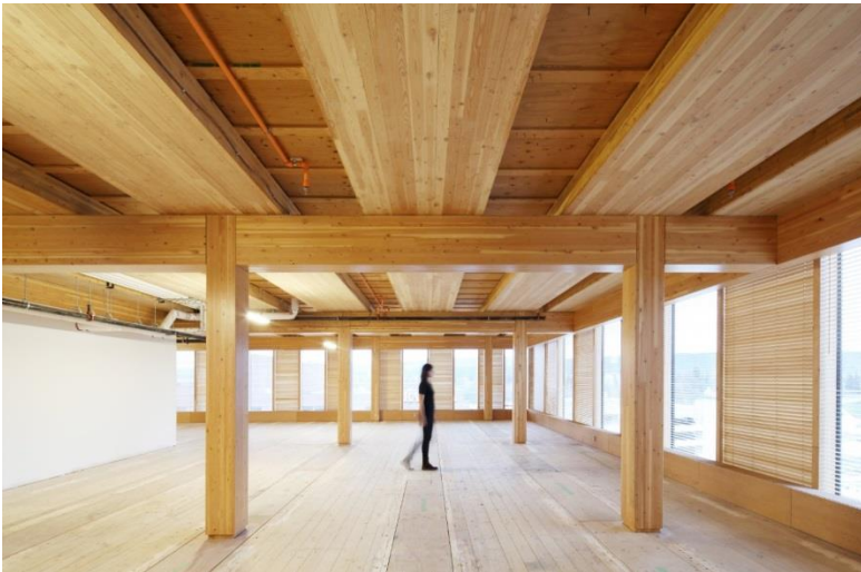
Figure 2 CLT beams within roof and floor assemblies at the Wood Innovation and Design Centre in Prince George (image courtesy: Michael Green Architecture).
