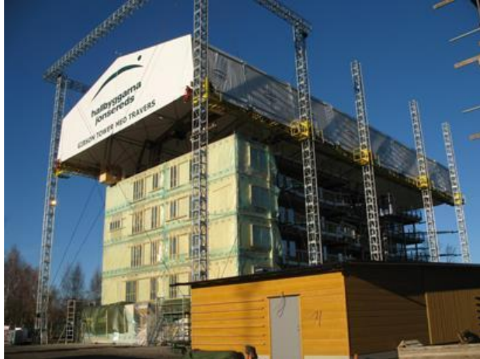
Figure 12 Using a liftable temporary roof to protect timber construction in Sweden.
