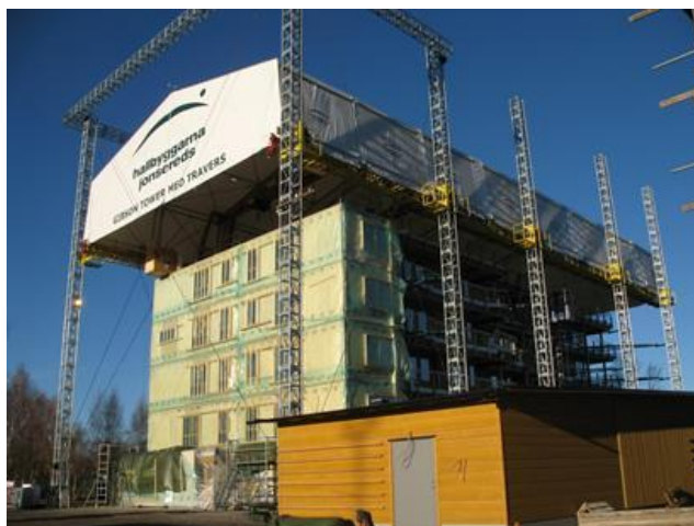
Figure 5 Using a movable tent to protect the entire construction in Sweden
