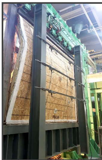
Standard fire resistance test of an exterior lightweight wood-frame wall assembly.
