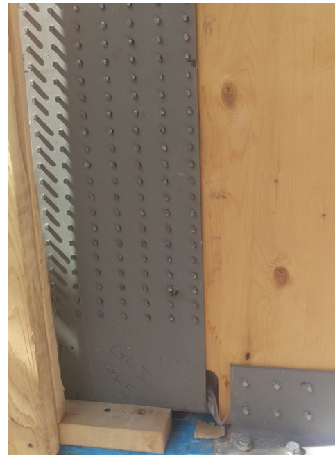
Flat strap drag strut and joint sealant tape. Images courtesy of Moses Structural Engineers
