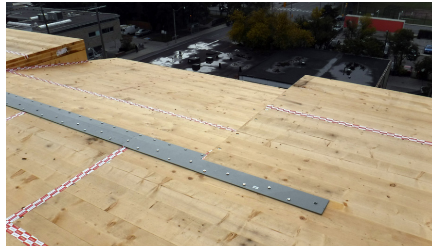
Flat strap drag strut and joint sealant tape. Images courtesy of Moses Structural Engineers
