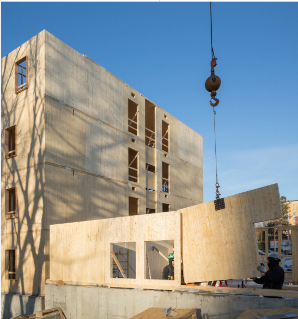
FIG 1: Open panel installation 70
