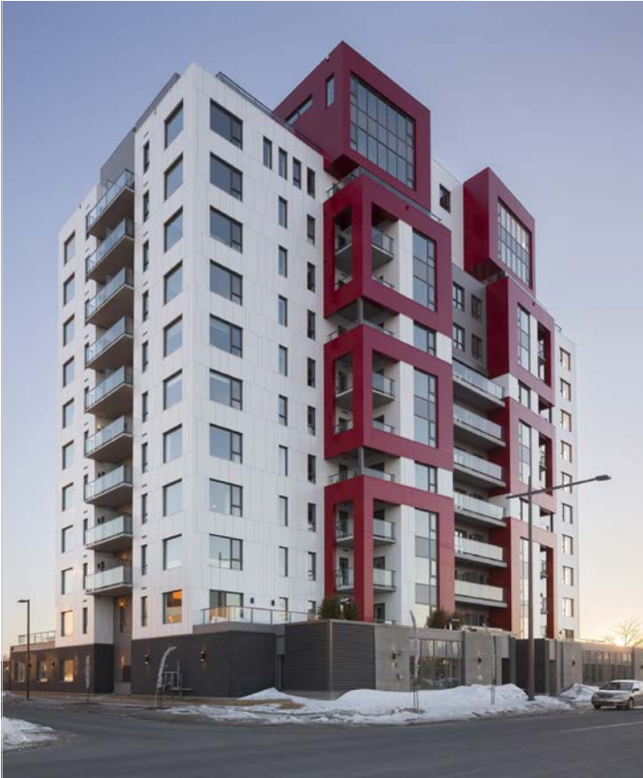
It took only four months, from December 2016 to April 2017, to erect the wooden structure of Quebec City's Origine: a 13 storey high, remarkable landmark and tallest wood building in eastern North America.
