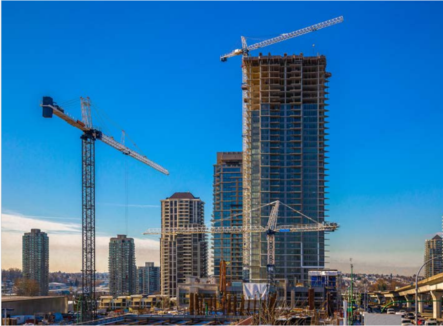
New construction of high-rise buildings in Burnaby, Vancouver
