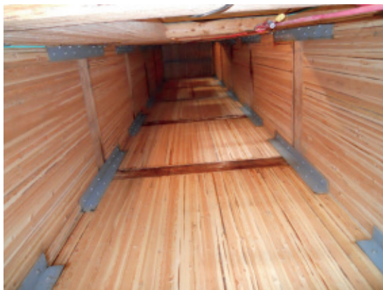
Figure 4.55: Example of a nail-laminated timber elevator hoistway.
