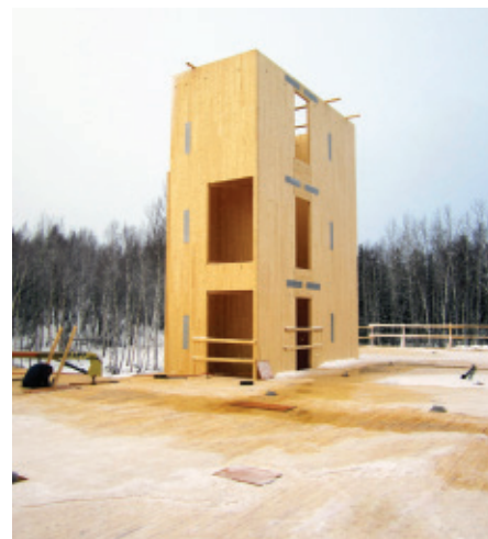
Figure 4.56: Example of an elevator hoistway composed of cross-laminated timber (CLT) solid panels.
