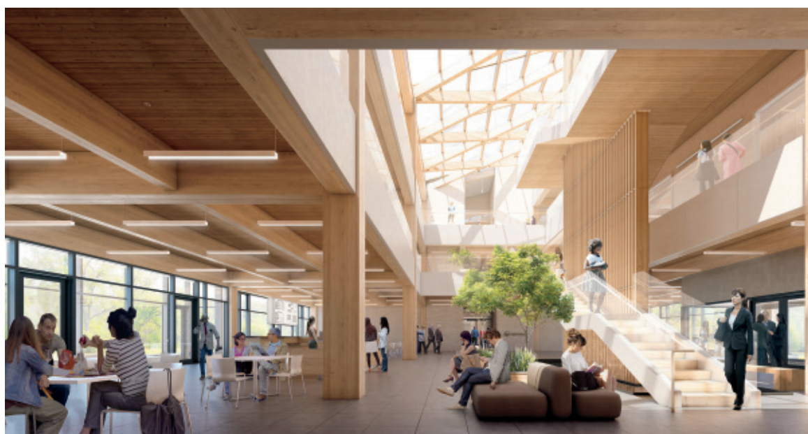
Figure 2.37: A proposed design for the new Ontario Secondary School Teachers' Federation architectural design by Moriyma & Teshima Architects, structural design by Fast + Epp. The building design utilizes a 9m x 9m mass timber-framed structural system consisting of deep girders in one direction and purlins in the other.
