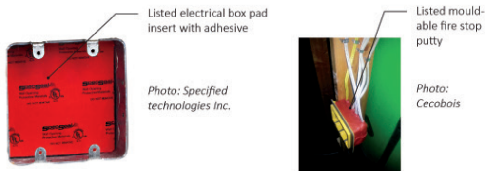
Figure 4.37: Examples of fire stops for electrical boxes.
