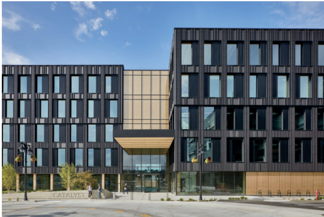
Figure 2.35: Catalyst Building by Michael Green Architecture. Photo by Benjamin Benschneider.
