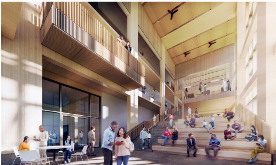
Figure 2.47: Limberlost Place (formerly The Arbour) at George Brown College, by Moriyama & Teshima Architects and Acton Ostry Architects, structural design by Fast + Epp. The building design utilizes the flat slab band cross-laminated timber structure with localized areas of composite concrete and CLT decking to manage the shear action.
