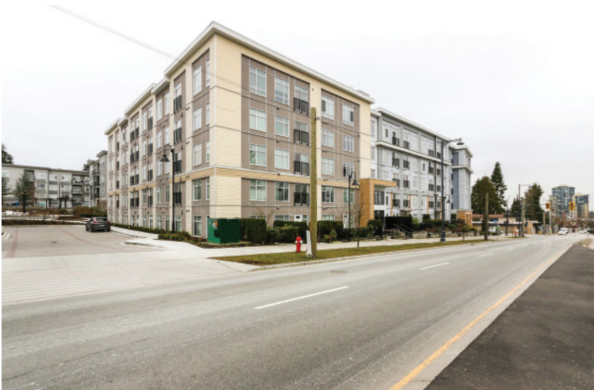
Figure 2.72: Quatro 3 in Surrey, B.C., completed in 2012 by Cotter Architects Inc.
