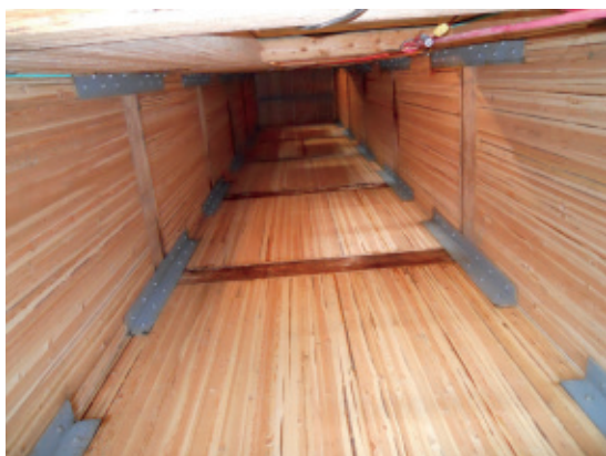
Figure 4.55: Example of a nail-laminated timber elevator hoistway.
