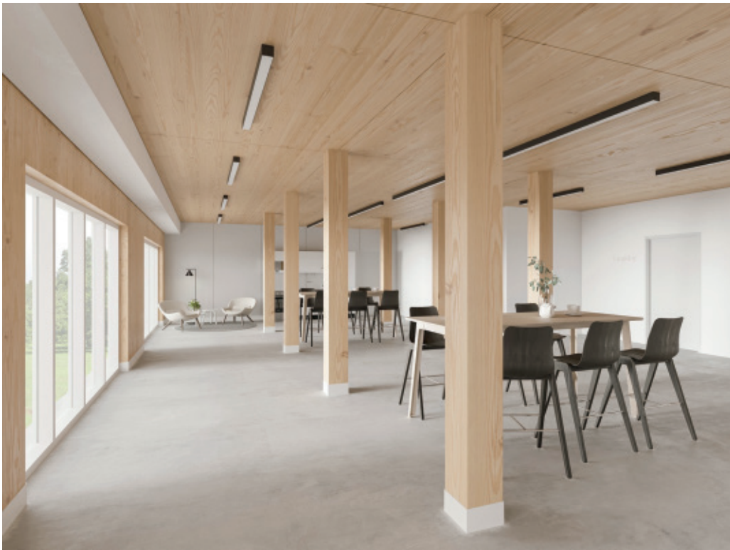
Figure 2.59: Concept rendering of the interior of the ground floor amenity space. The structural grid in this location shifts from a panelized system to a post and panel system. Image Source: Edge Architects and Element5.
