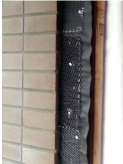
Figure 6.04: Thin brick veneer.
