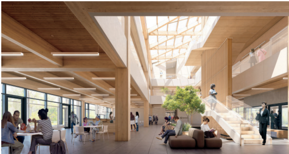
Figure 2.37: A proposed design for the new Ontario Secondary School Teachers' Federation architectural design by Moriyama & Teshima Architects, structural design by Fast + Epp. The building design utilizes a 9m x 9m mass timber-framed structural system consisting of deep girders in one direction and purlins in the other.
