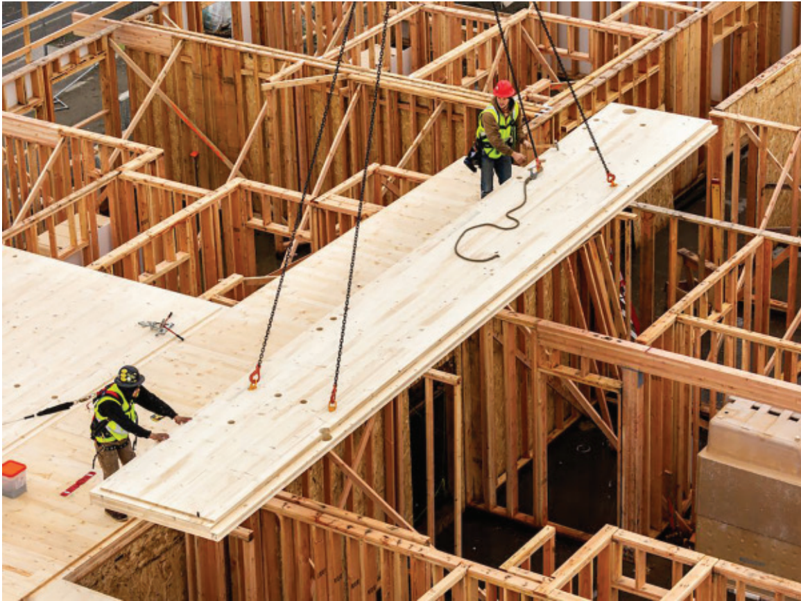
Figure 2.65: Example of platform framing using cross-laminated timber (CLT) as the floor slab and lightweight wood-framing load-bearing walls below for a residential project. The off-site prefabrication of CLT can offer acceleration of on site construction timing.
