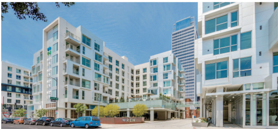
Figure 2.28: Wren multi-family complex in southern California by Togawa Smith Martin.
