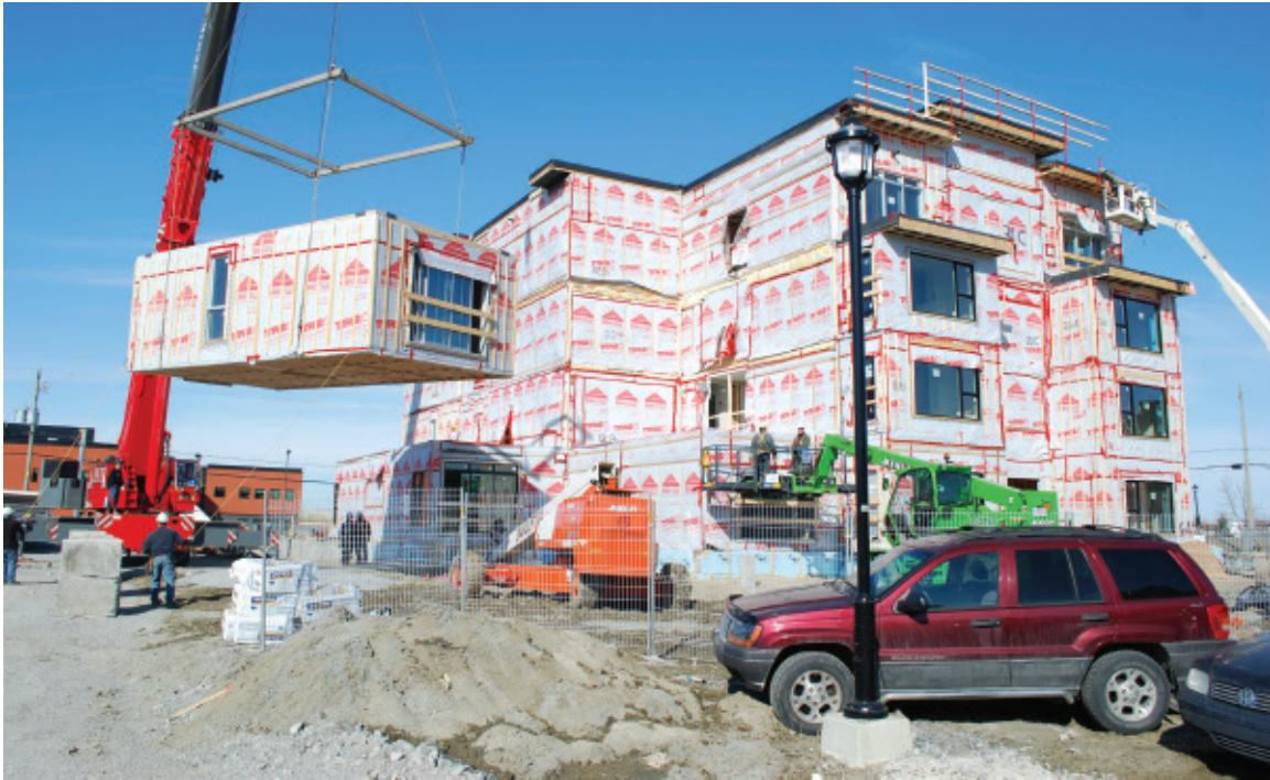
Figure 7.9: Volumetric modular construction. Image courtesy of Bonneville Industries.
