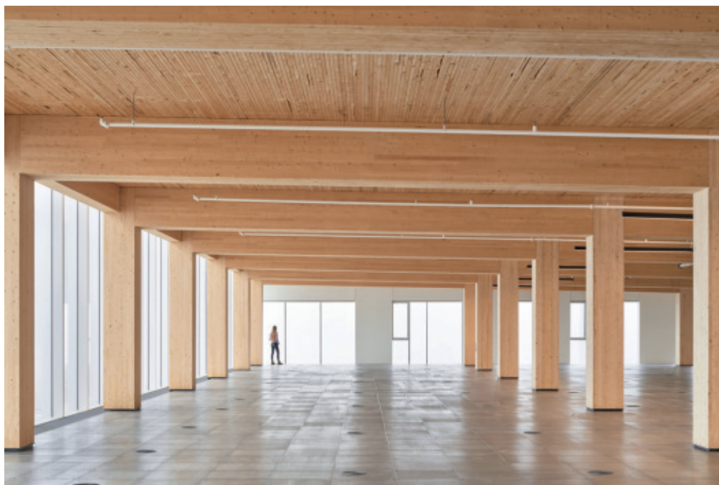
Figure 2.41: The interior of 80 Atlantic Avenue in Toronto, Ontario. Architectural designed by BPN Quadrangle (formerly Quadrangle Architects Ltd.), structural design by RJC for Hullmark. The method utilizes a framed mass timber structure of approximately 8m x 8m consisting of deep girders in one direction and a short deck in the other, freeing the structure of intermediate purlins.
