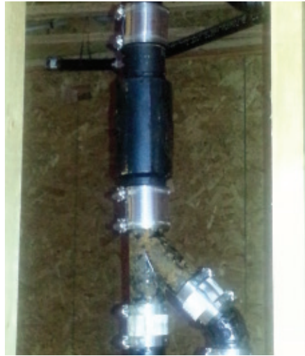
Figure 5.01: Pipe sleeves accommodating shrinkage.
