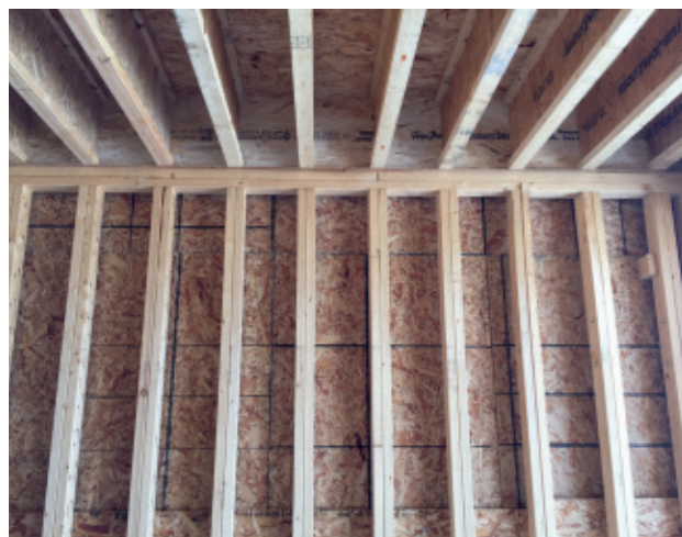
Examples of factory-built systems in use: Wall panels and floor systems. Installation is rapid. Images courtesy of Steven Street.
