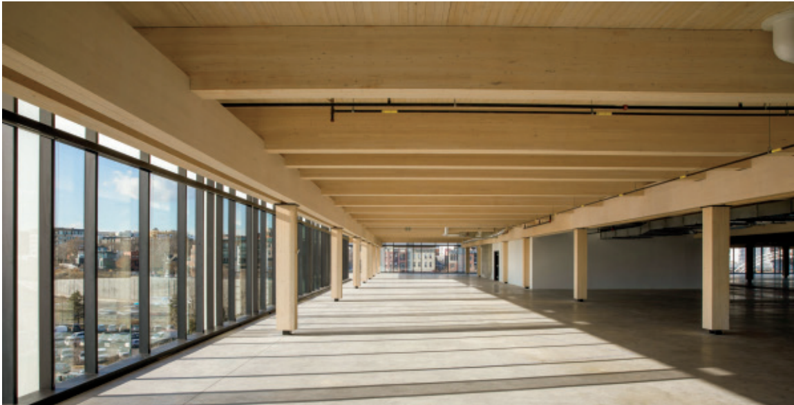
Figure 2.38: Platte Fifteen in Denver is a five-storey office structure that utilizes the 30'x30' (9.1m x 9.1m) optimal bay to optimize structural spans of the mass timber component. The purlins are notched and into the girders, leaving a gap above for the running of services.
