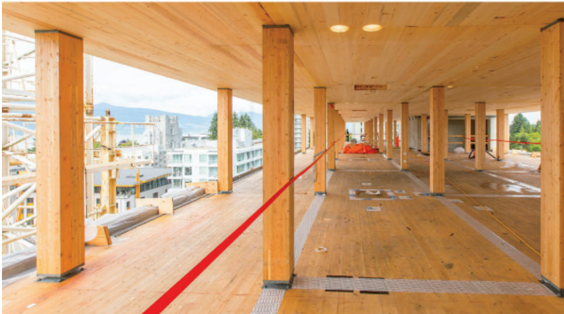
Figure 2.43: Brock Commons Tallwood House architectural design by Acton Ostry Architects, structural design by Fast+Epp illustrating a short span CLT floor structure point loaded on glulam columns.
