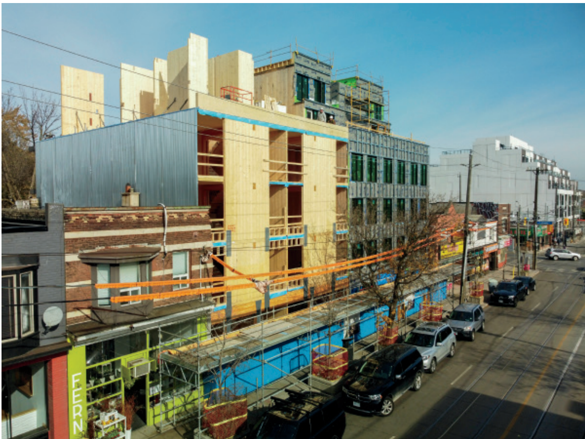
Figure 2.55: View during construction from Queen Street East.
