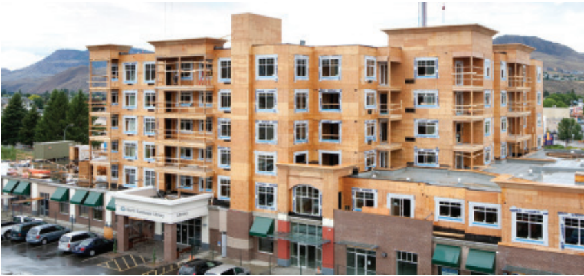
Figure 2.67: Construction at Library Square, Kamloops, B.C. Credit: Stephanie Tracey.
