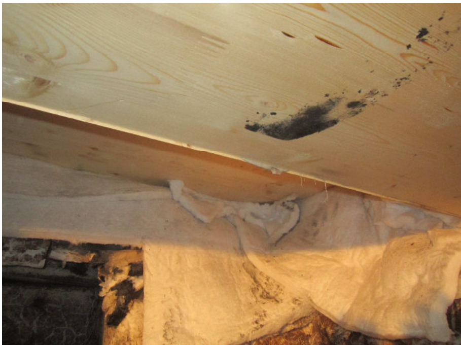
Exposed Side Prior to the Fire Test
