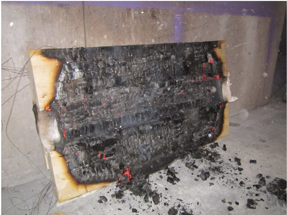
Exposed Side After the Fire Test
