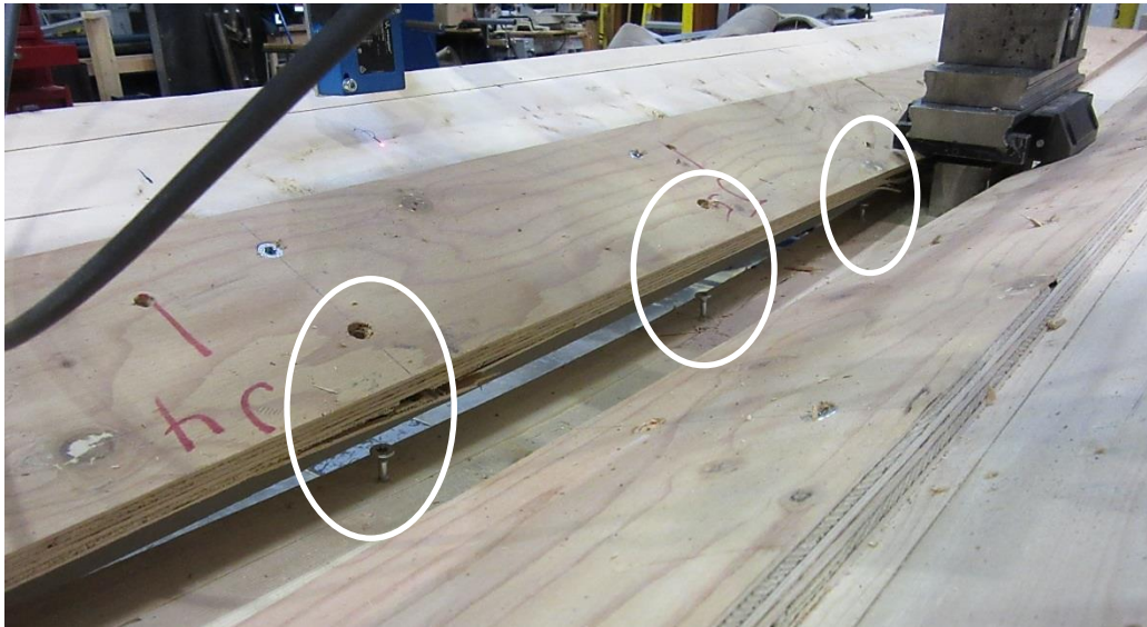
Figure 5. Head pull-through in CLT bending test under ambient conditions
