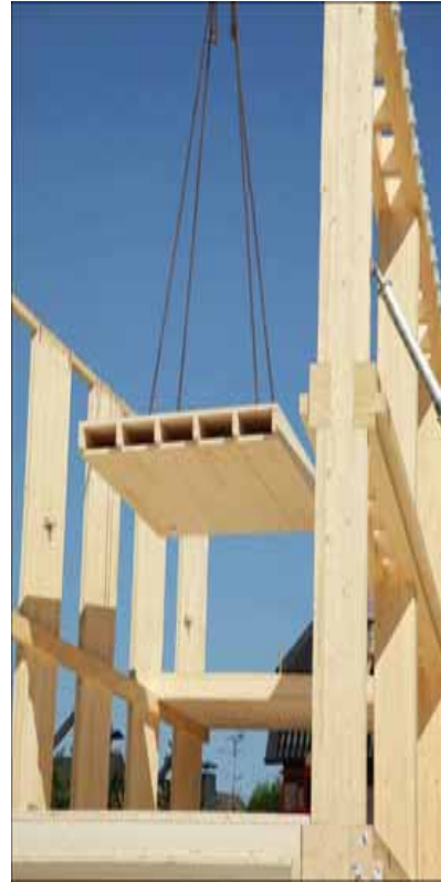
Hollow Box floor system 7.5m span, 40cm thick
