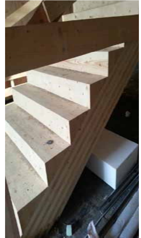
Prefabbed elements for faster installation
