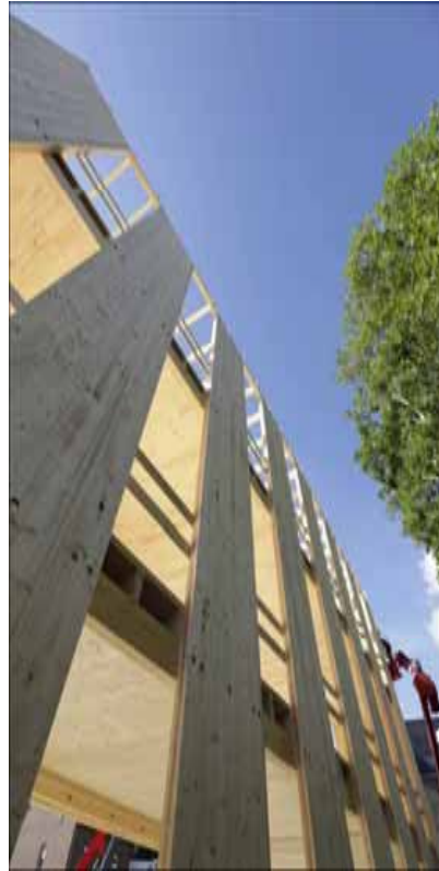
3 Level X-Lam walls 10.795m tall. Assembled on sawhorses then tilted into place
