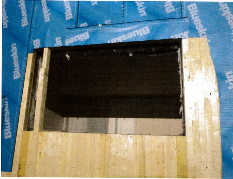
Figure 4. Wall system under construction.
