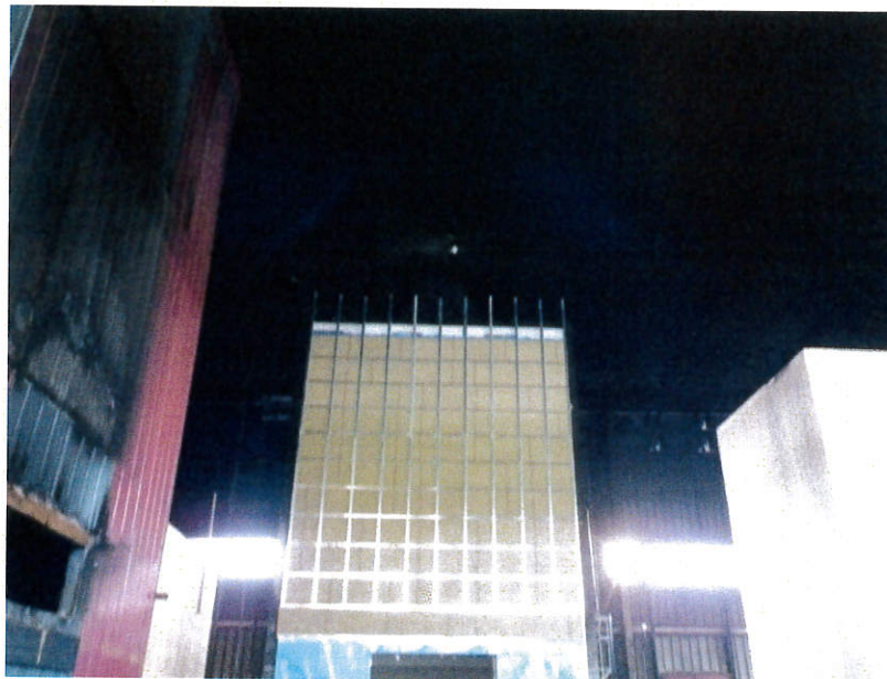
Figure 5. Installation of Roxul insulation.
