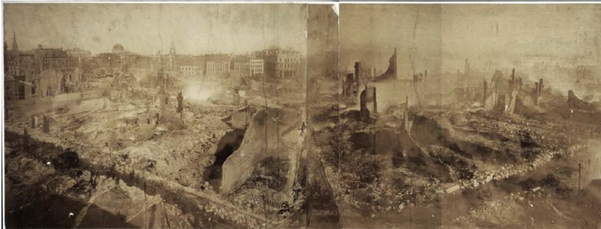
Figure 3: A mosaic photograph showing the destruction in Boston following the fire.
