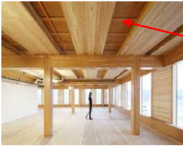
Plywood furring used to create an air space between plywood roof sheathing and CLT panels
