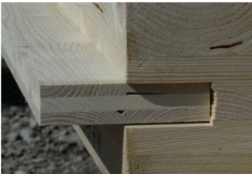
Figure 4.6. Example wall to wall panel connection (Photo: D. Moses).
