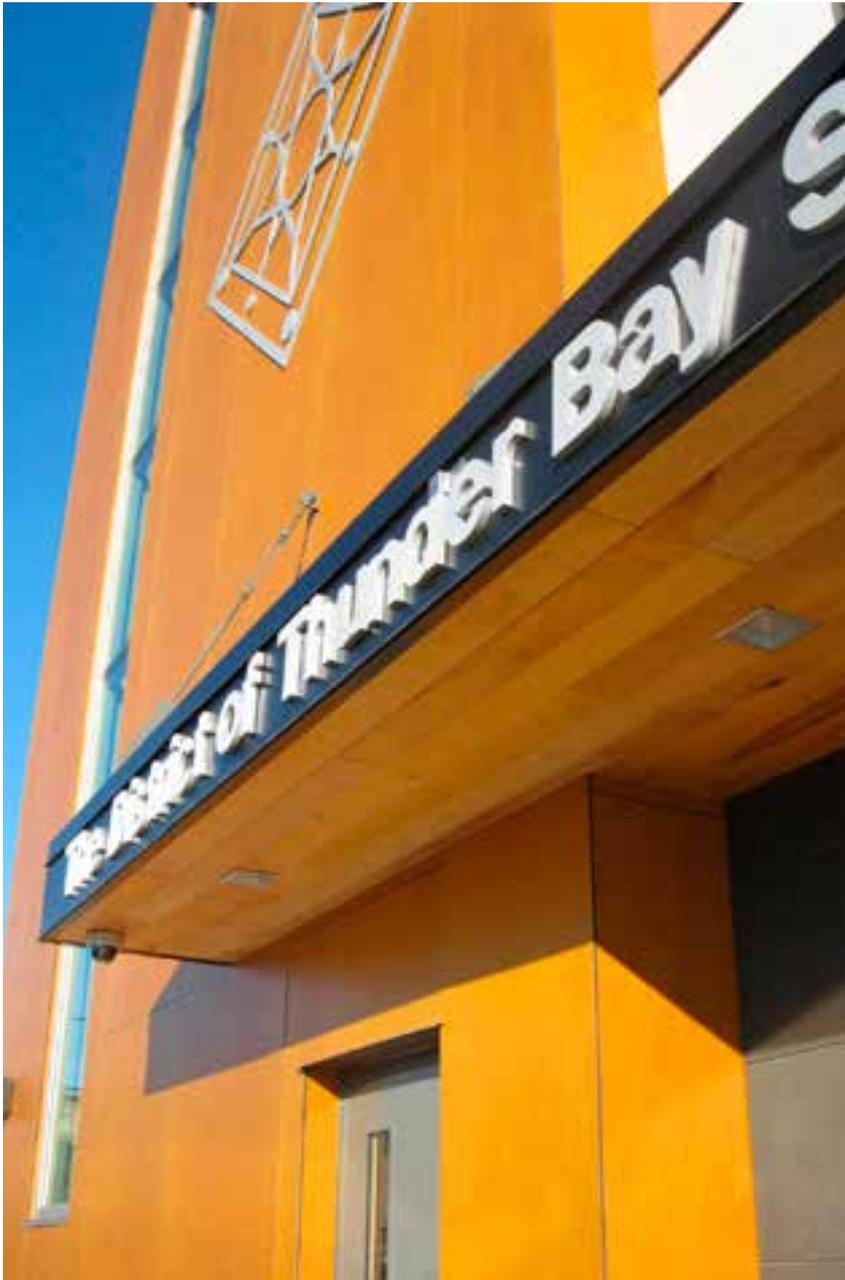
The relatively light weight of the wood superstructure reduced foundation costs compared to what would have been required for a concrete or steel superstructure. A high water table did not permit below grade parking on the site so parking is provided on an adjacent lot.
