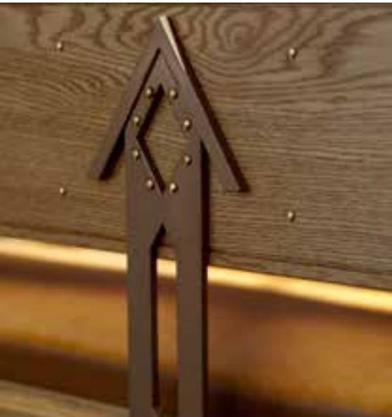
**R**io Roca Chapel is located along the Brazos River in Texas. The 1,080-sq.ft. chapel is used for private services. The chapel is constructed of stone, glass, steel and wood, and utilizes tension bars, with turnbuckles at each of the bars, to provide bracing for the glass walls and copper roof. The structure is a series of custom-designed steel and wood fitch systems with fir tongue and groove decking above.
