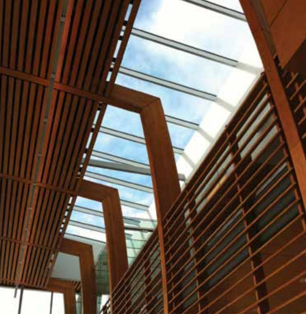
an initial wood impression to passengers who must walk underneath the suspended structure while being processed by Canada Customs. Proceeding to the welcome center, passengers are surrounded by the main structure consisting of curved and straight Douglas fir glulam columns and beams, and Douglas fir wood slat screens. These elements give a sense of enclosure, warmth and directionality, and open up the space to the view of the harbor beyond.
