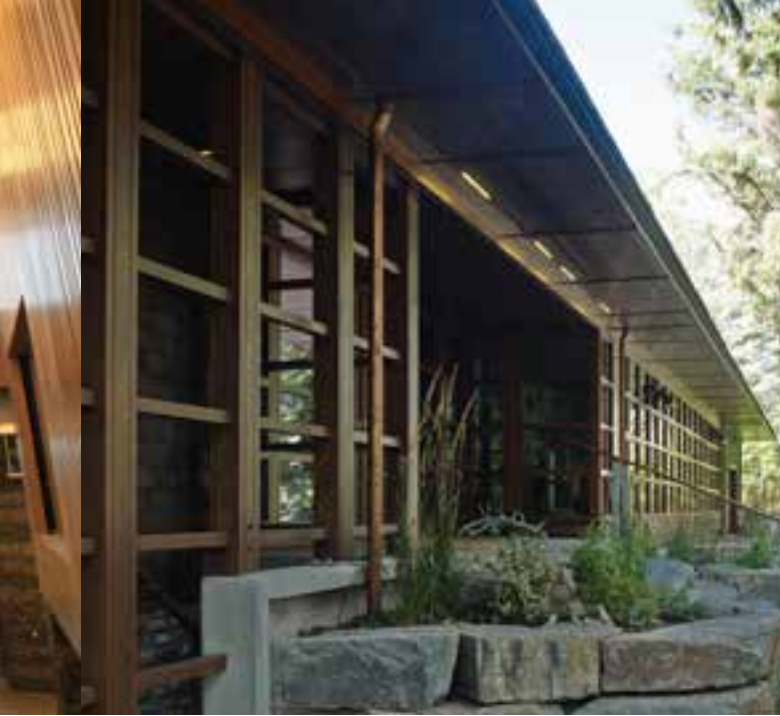
Mountain House, Alberta | Sturgess Architecture Photo by Kai Mushens Photography
