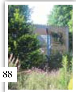
JC Raulston Arboretum Lath House
