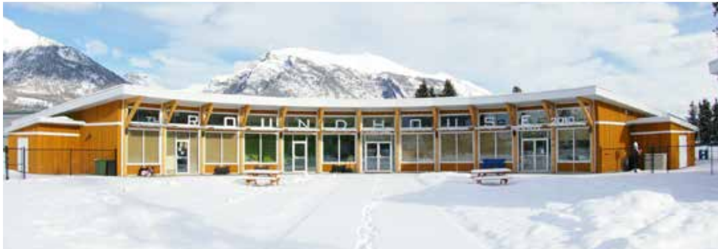
Roundhouse Daycare and Preschool, Canmore, AB Lloyd R McLean Architect with russell and russell design studios | Photo by Alasdair Russell
