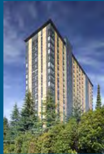
Wood Innovation Award Brock Commons Tallwood House Vancouver, BC Please see page 140
